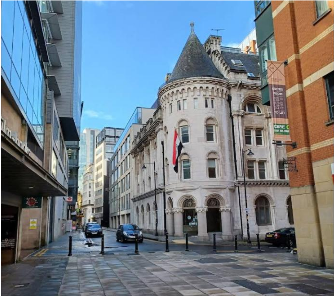
(Figure 12: Barclay's building adjacent to proposed application site)
