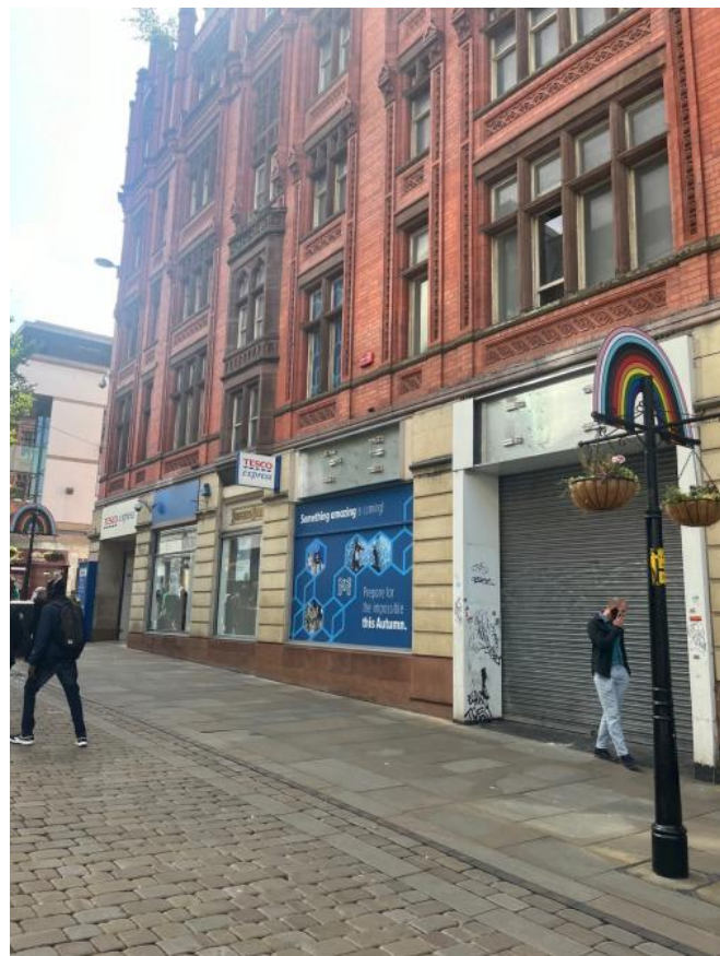
(Figure 12: Non-designated 58-66 Market Street)
