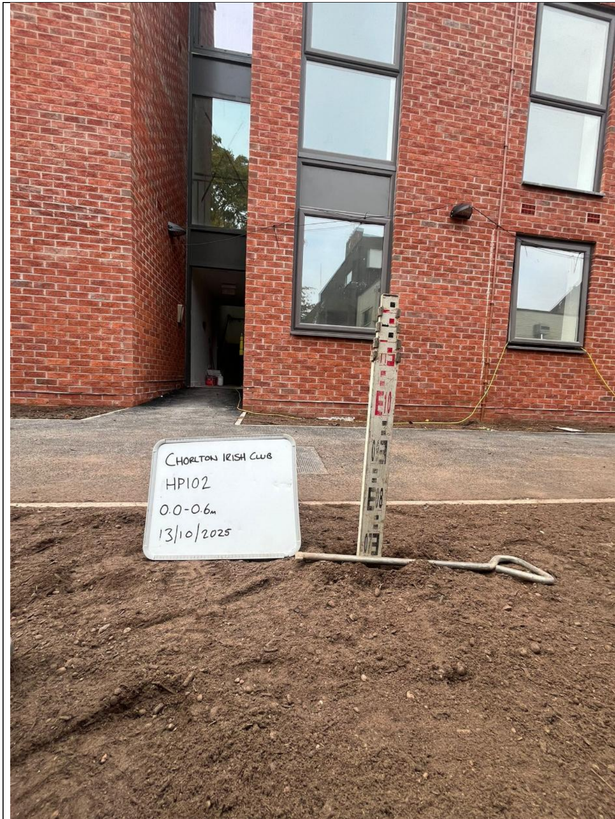
Plate 6: View showing depth of cover on HDP102.
