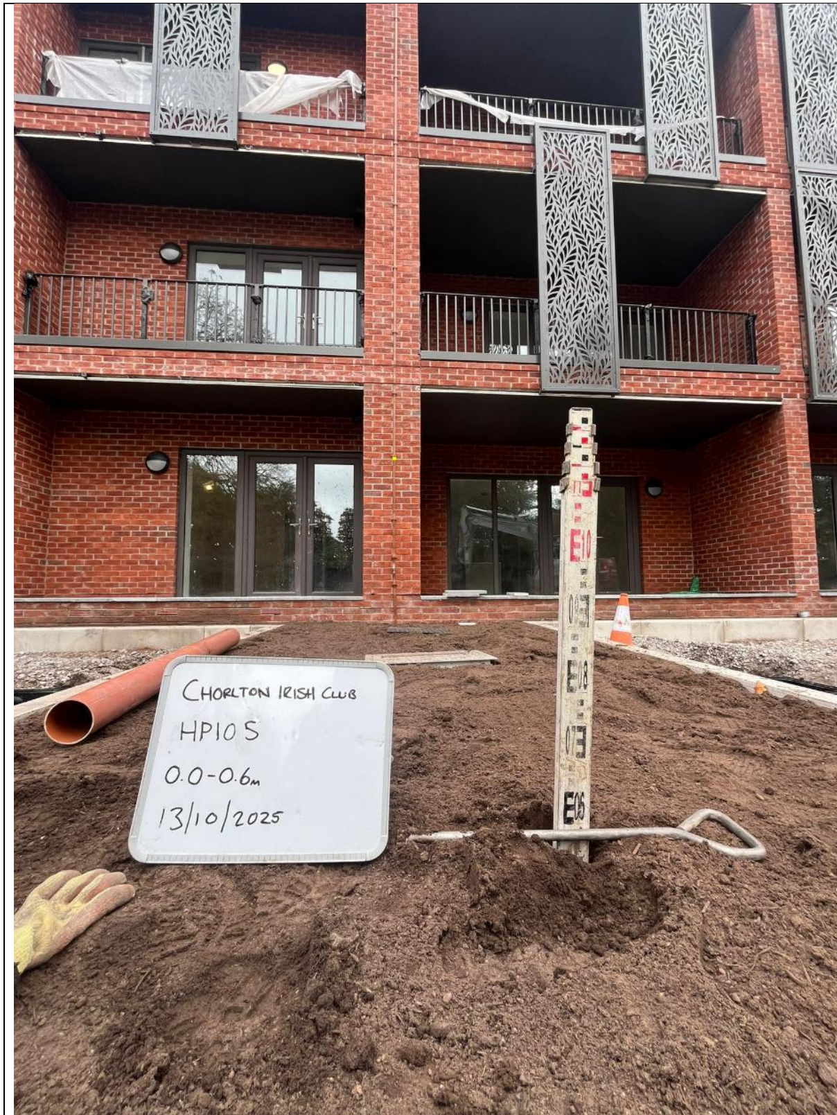
Plate 15: View showing depth of cover on HDP105.
