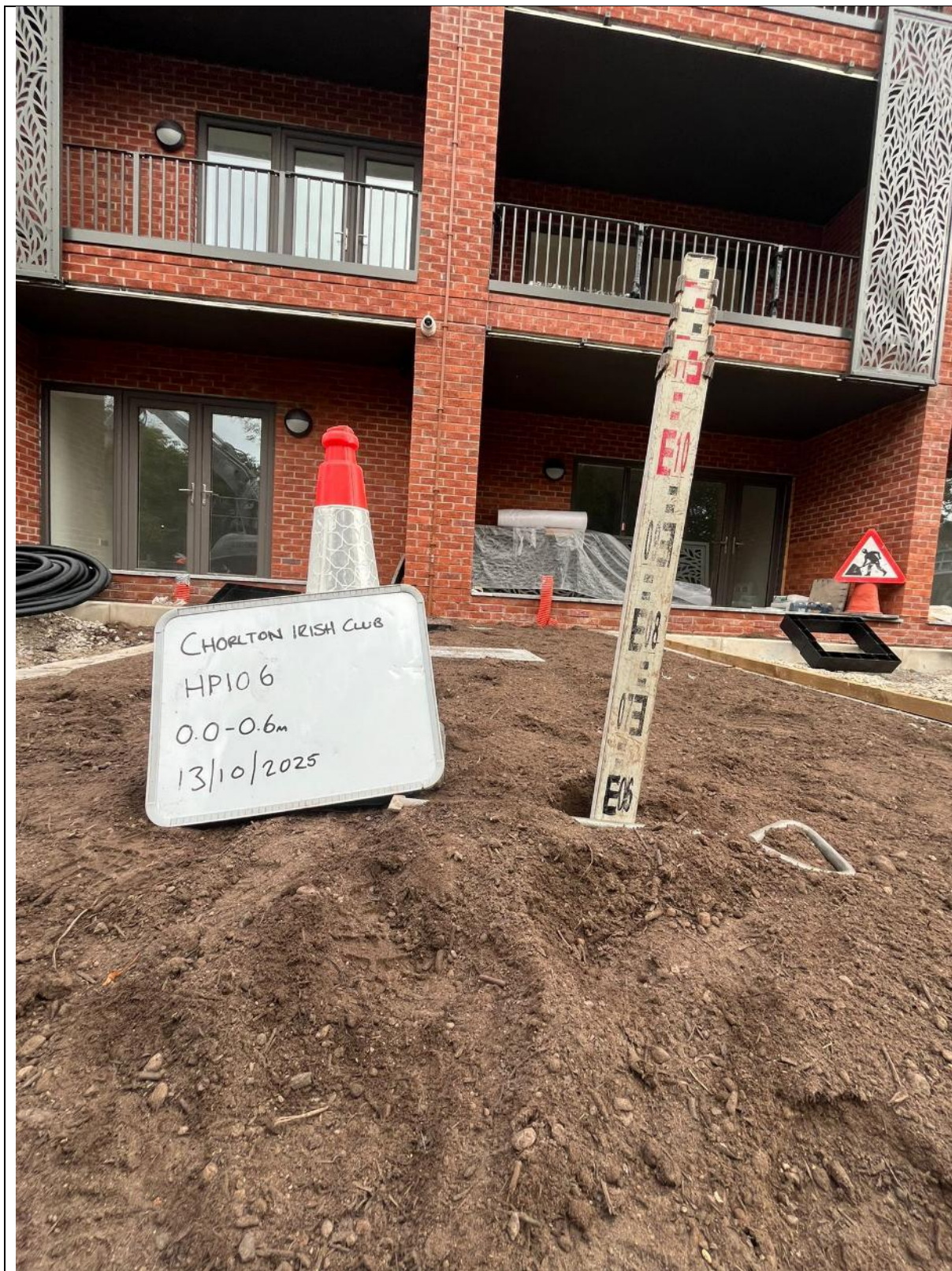
Plate 18: View showing depth of cover on HDP106.
