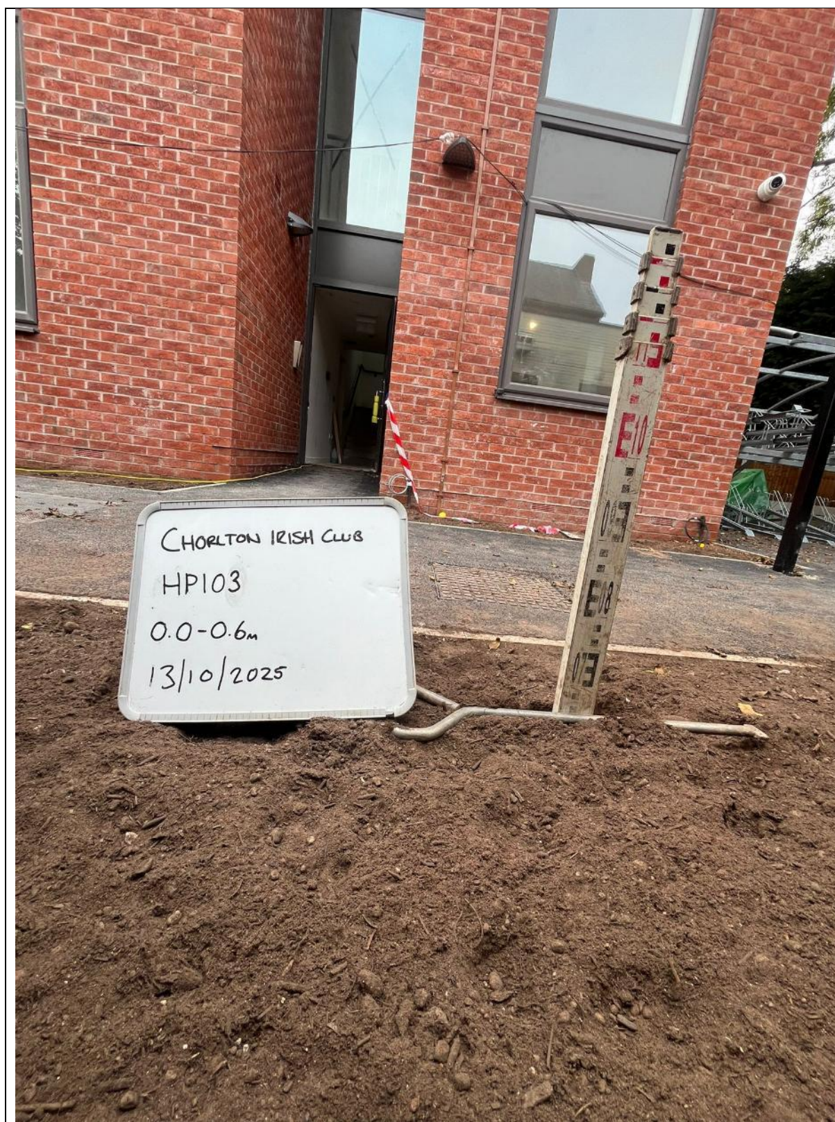
Plate 9: View showing depth of cover on HDP103.
