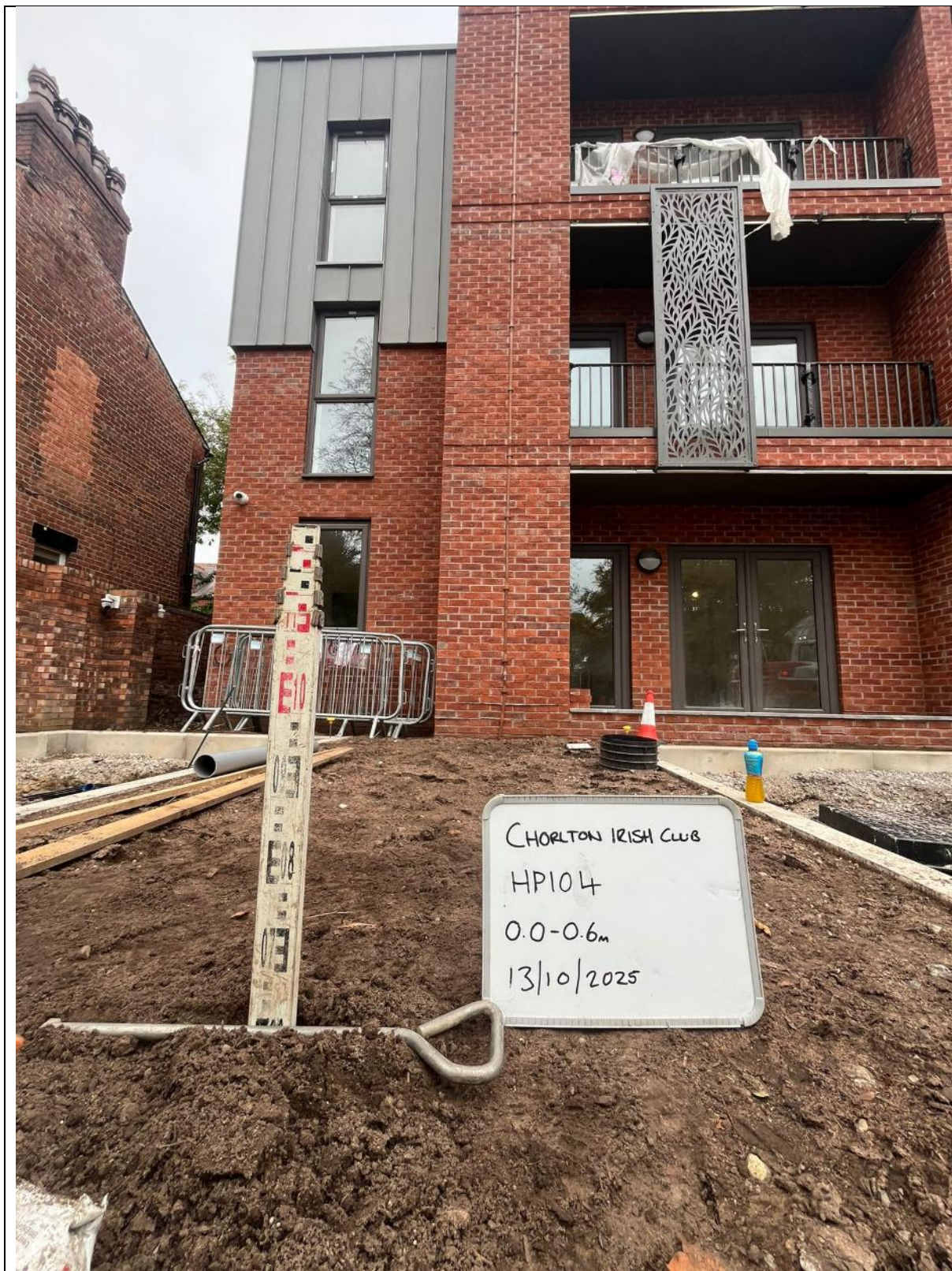
Plate 12: View showing depth of cover on HDP104.
