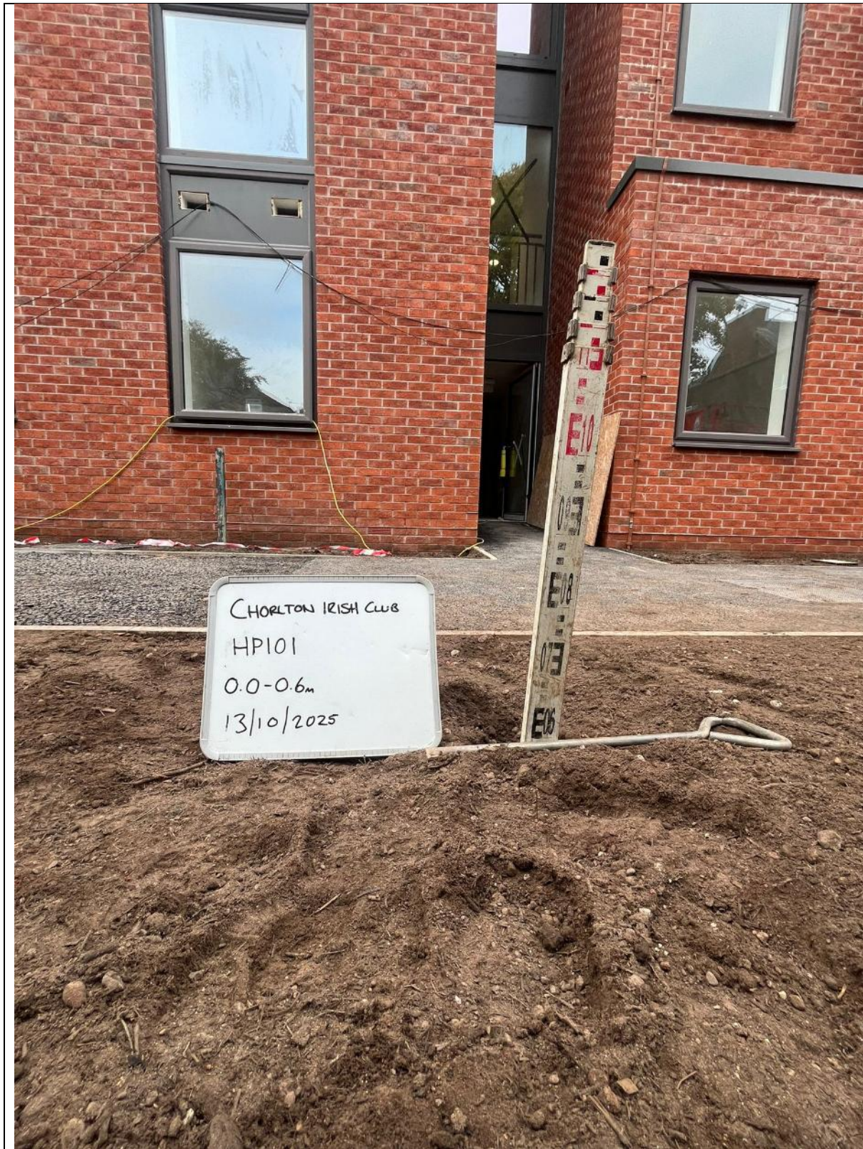
Plate 3: View showing depth of cover on HDP101.
