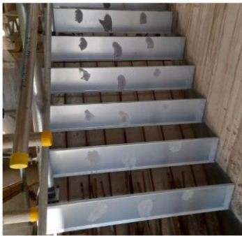
Figure 12 - Stair Master: Perm Shutters, Metal Risers, Preloaded Rebar
