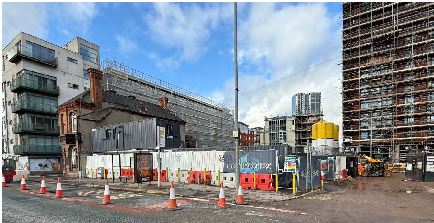
Plate 7: View of hoarded Site, showing demolished former gas works warehouse, looking north-west from Rochdale Road
