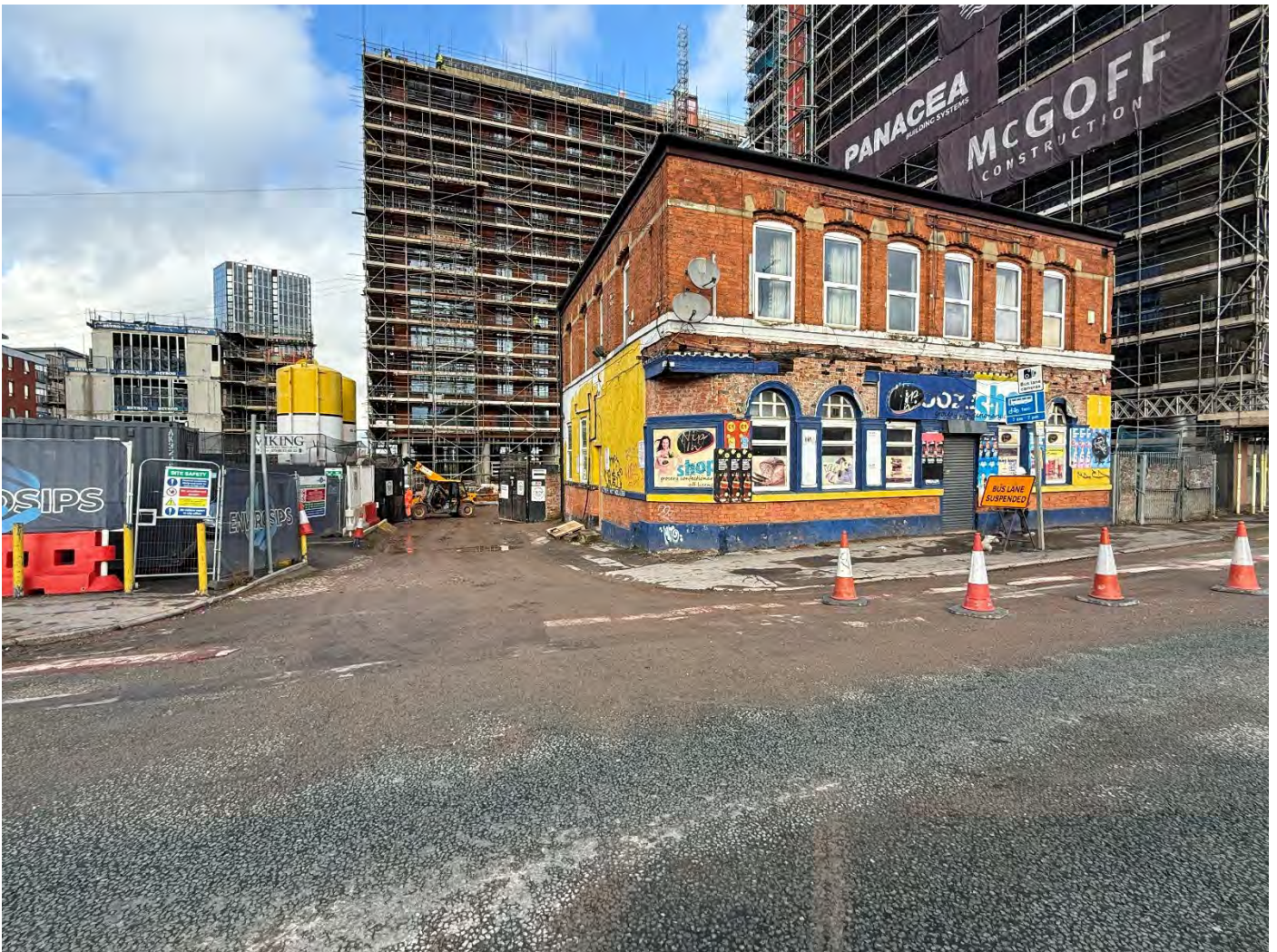
Plate 6: View of south-facing elevation of the former Victoria Inn, looking broadly north-east
