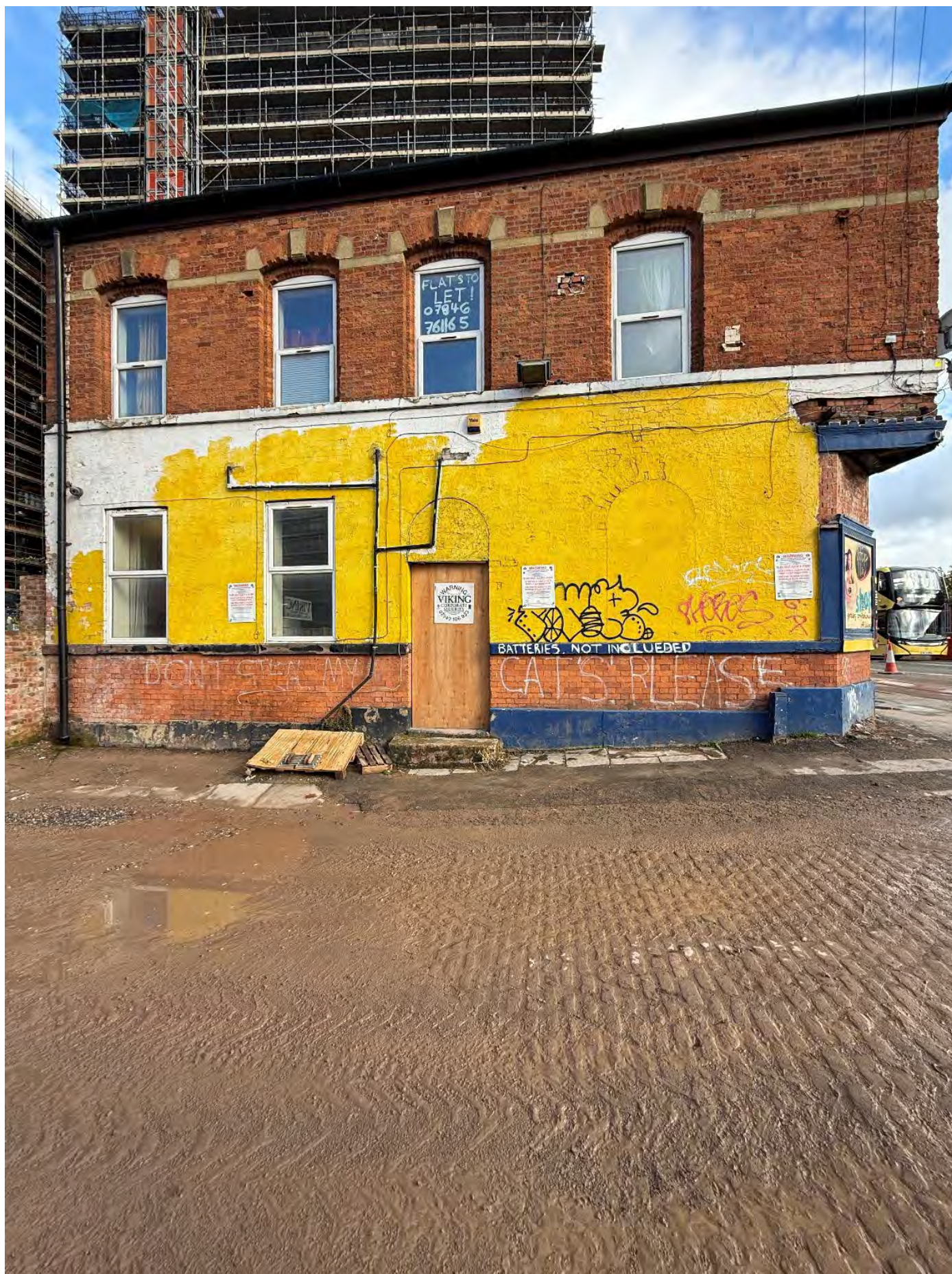
Plate 9: View of east-facing elevation of the former Victoria Inn and stone sett road surface of Ashley Street, looking east
