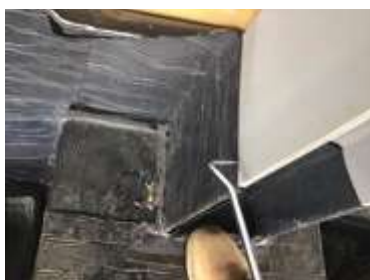
Probe testing stanchion sealing
