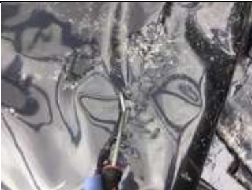
Testing sealed hand welded membrane lap joint
