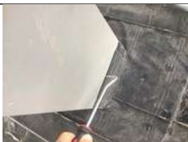
Probe testing stanchion detailing
