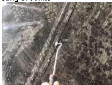
Testing auto welded membrane lap joint
