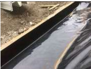
Membrane extended up the perimeter temporary shuttering
