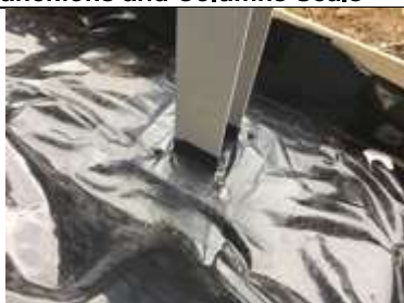
Sealed stanchion detailing
