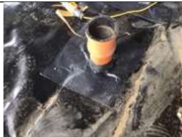
Sealed pipe penetrations
