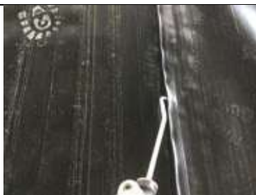
Pick testing along the auto welded lap joint within Pour area 5.
