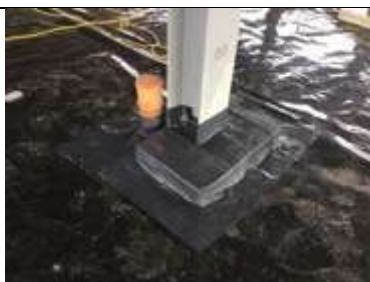
Steel stanchion detailing sealed within pour area 5.
