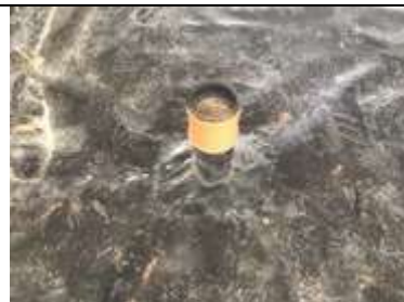
Sealed pipe penetration
