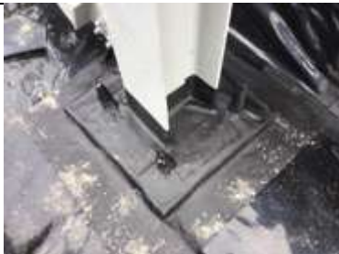
Stanchion detailing sealed using Juta GP1 SAM and heat applied
