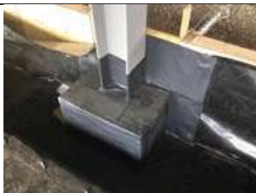
Sealed internal stanchion and concrete surround detailing
