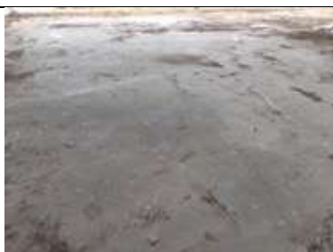
Sand blinded well rolled and compacted
