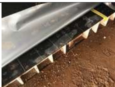
Heave board installed which the membrane is installed above
