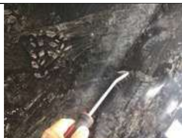
Testing hand welded membrane lap joint
