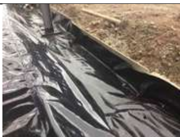
Perimeter membrane extended up the shuttering
