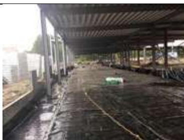
Pour 3 overview of completed works
