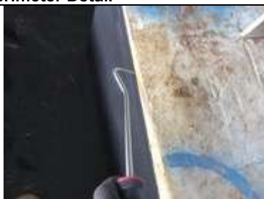
Internal perimeter concrete column retro fit detail testing
