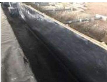
Membrane extended up the internal perimeter shuttering
