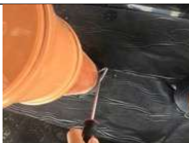
Probe testing pipe sealing
