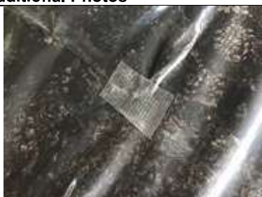
Defect repaired sealed using Juta GP1 SAM
