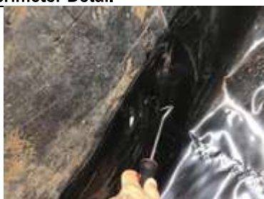
Testing perimeter hand weld
