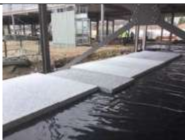
Insulation installed after the inspection
