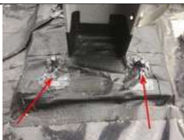
Butyl tape used to seal bolts
