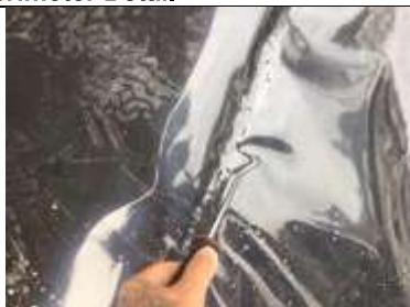
Testing perimeter membrane hand welded lap joint
