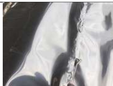
Pick testing carried out along the hand welded lap joint to pour area 5.
