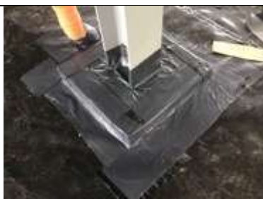
Sealed stanchion detailing
