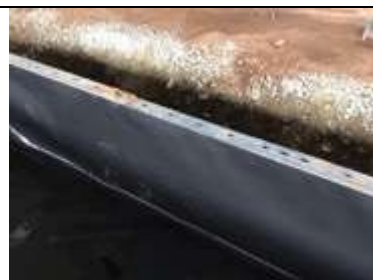
Membrane extended up the perimeter shuttering
