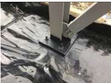
Sealed stanchion detailing
