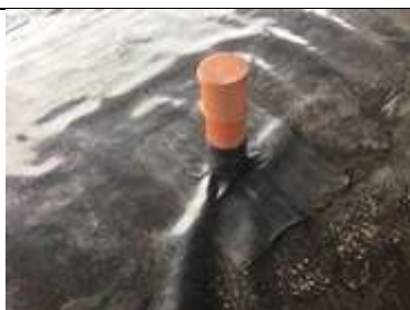
Sealed pipe penetration
