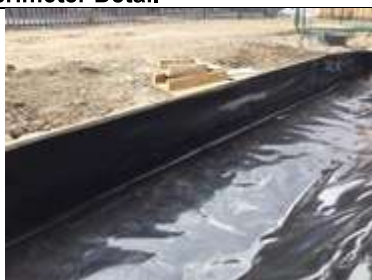
Membrane turned up the perimeter shutter and stapled at the top into place.
