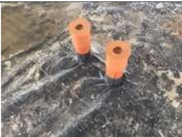
Sealed pipe penetrations
