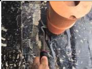
Testing pipe seals
