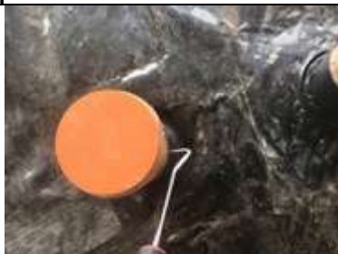
Probe testing pipe sealing
