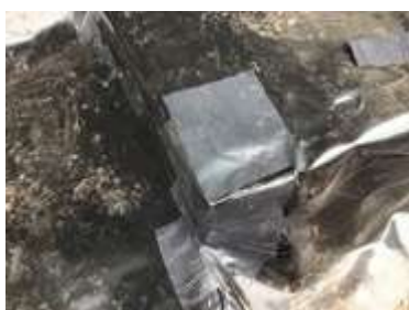
Sealed corner detailing
