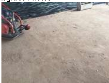
Blinding prior to the membrane installation
