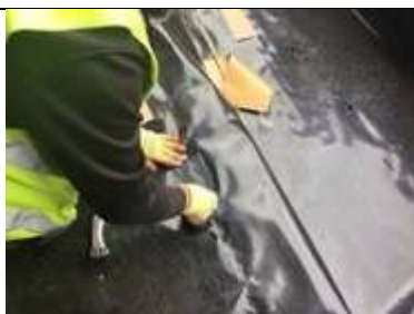
Installer repairing weld defect during the inspection
