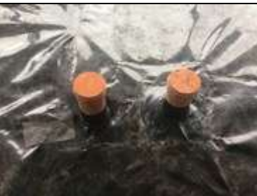
Sealed pipe penetrations
