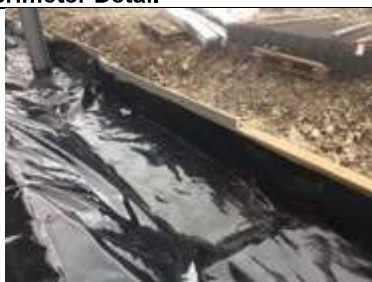
Perimeter membrane extended up the shuttering
