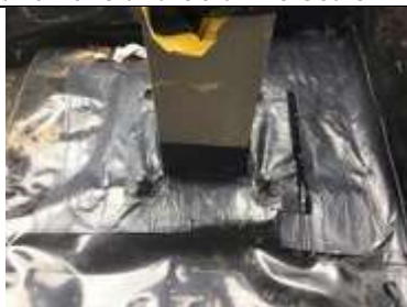
Sealed stanchion detailing
