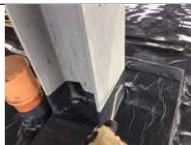
Pick testing to the stanchion detail within pour area 5.
