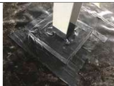
Sealed stanchion detailing
