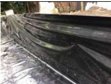
Perimeter membrane extended over the temporary shuttering
