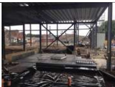
Remaining area of pour 3 yet to be installed
