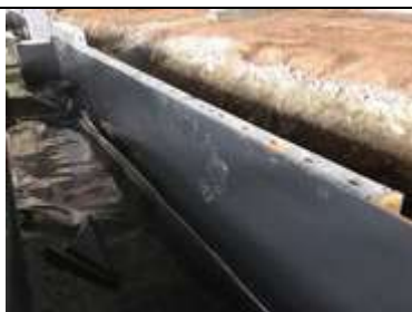
Membrane extended up the perimeter shuttering
