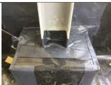
Sealed steel stanchion detail within pour area 3.
