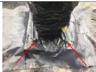
Double sided butyl tape used on the stanchion bolts
