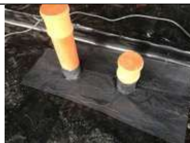
Sealed pipe penetrations
