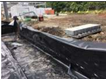
Perimeter membrane extended over the temporary shuttering
