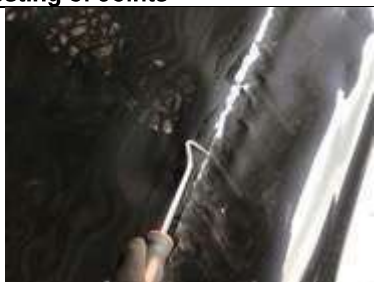
Testing sealed hand welded membrane lap joint
