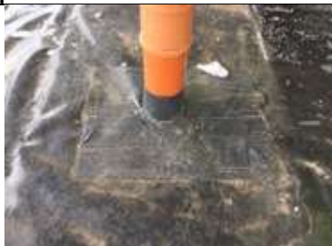
Sealed pipe penetration detail within pour area 3.
