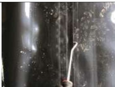
Testing sealed auto welded membrane lap joint
