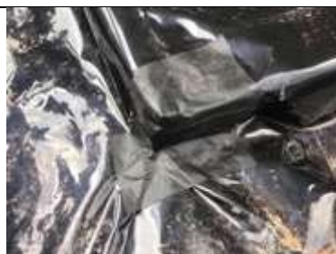
Corner detailing sealed sealed using Juta GP1 SAM
