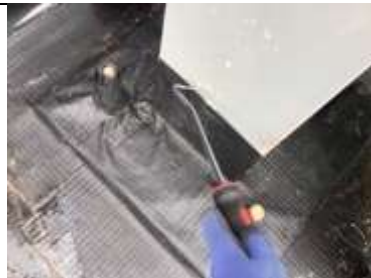
Pick testing stanchion sealing
