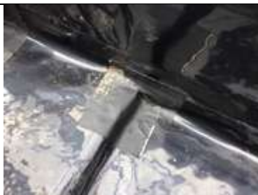
Corner detailing sealed using Juta GP1 SAM and heat applied
