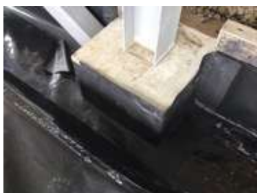
Stanchion concrete surround sealed sealed using Juta GP1 SAM
