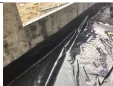
Membrane extended up the outer perimeter shuttering
