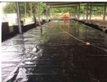
Alternate overview of the pour area installed
