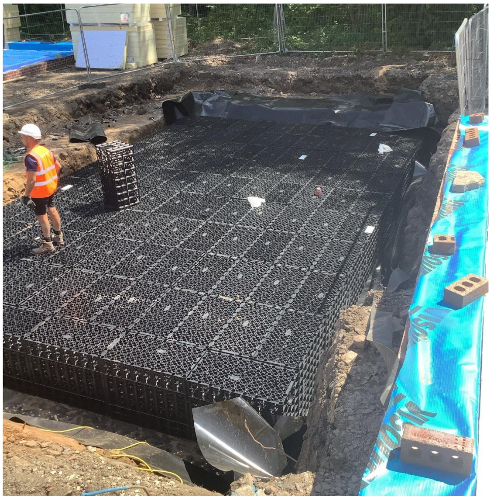
Installation of cellular attenuation
