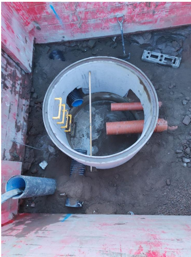
Internal Manhole Benching
