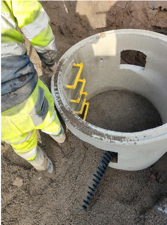
PCC Manhole Ring and Step Irons
