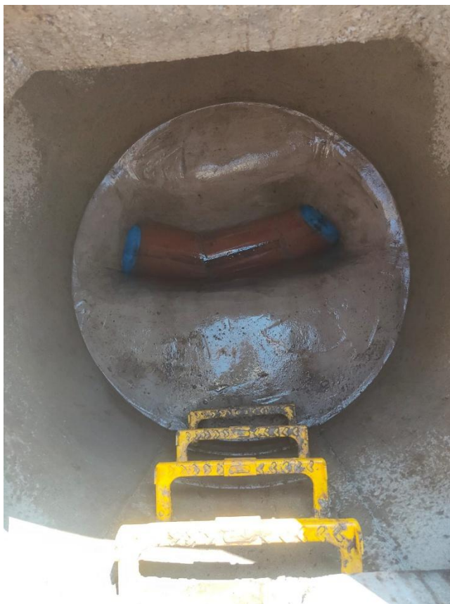
Internal Manhole Benching
