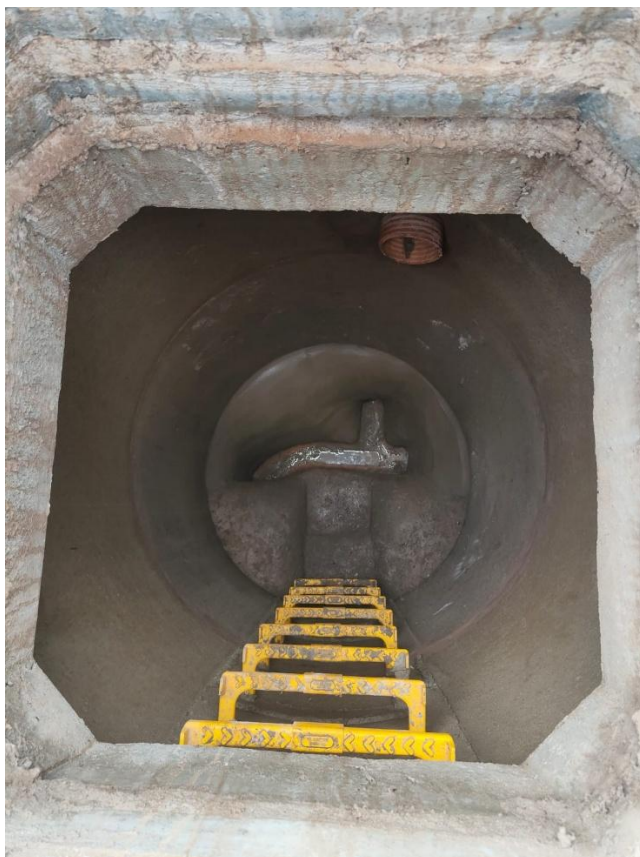
Internal Manhole Benching
