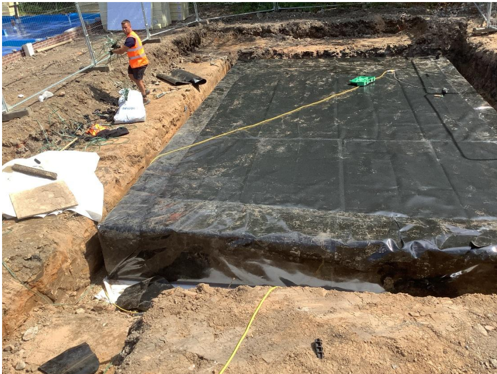
Installation of impermeable wrapping
