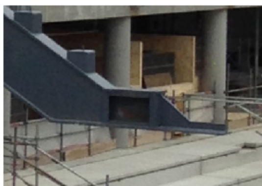
Figure 3-3 - Indicative steel raker tip
