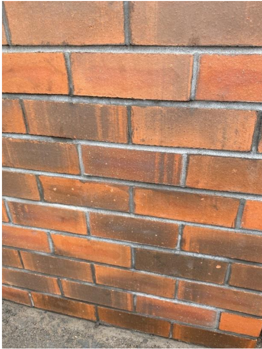
Figure 3: Close up brick 19.09.26
