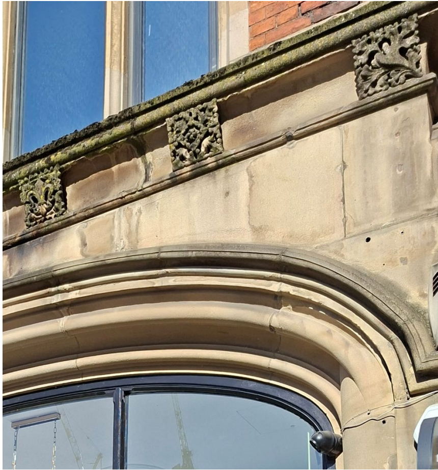
Fig 3: Photo showing existing fixing holes (filled) between the hood moulding of the arch and string course over. These appear to be of various dates and are evidence of previous awnings fixed to the building in this location.
