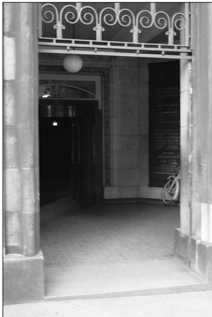
Figure 23 - Photograph dating to 1958, showing the original lobby.
