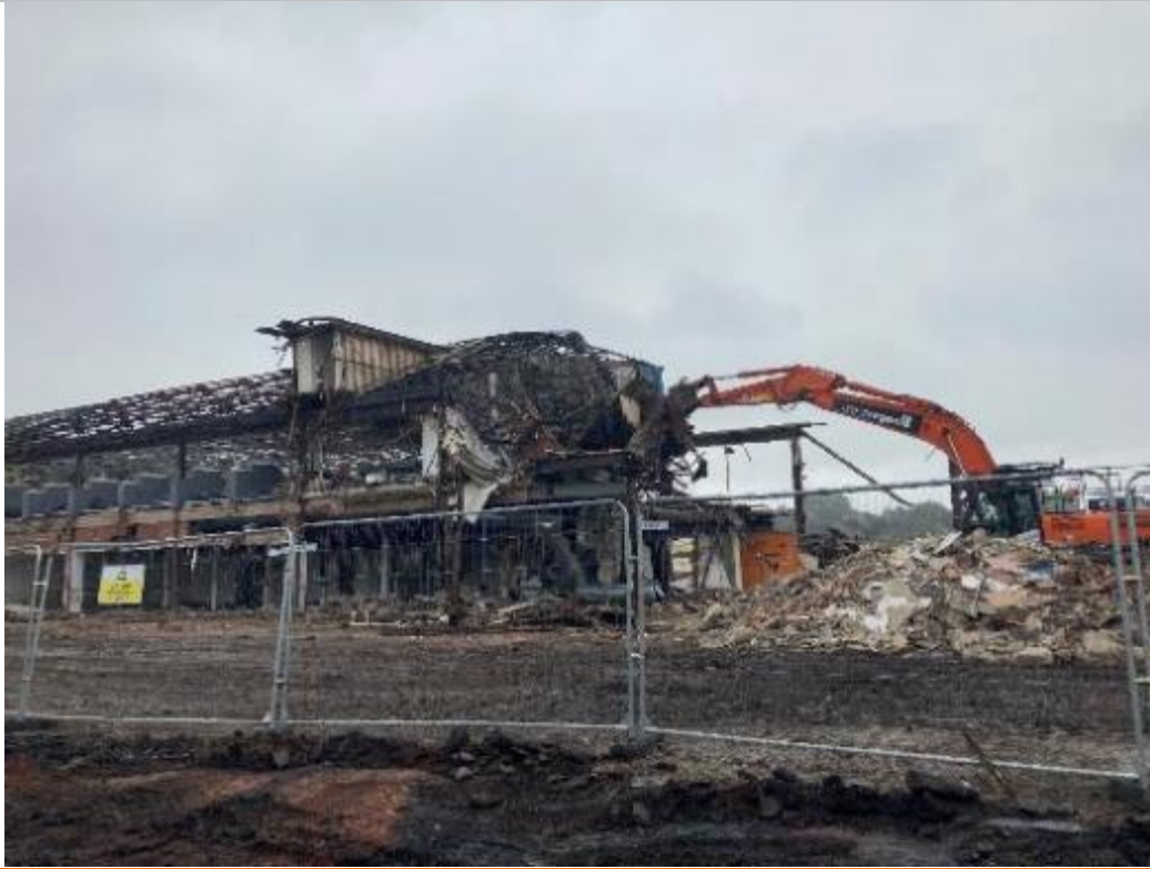
PLATE 7 SITE CLEARANCE- DEMOLITION OF EXSISTING BUILDINGS
