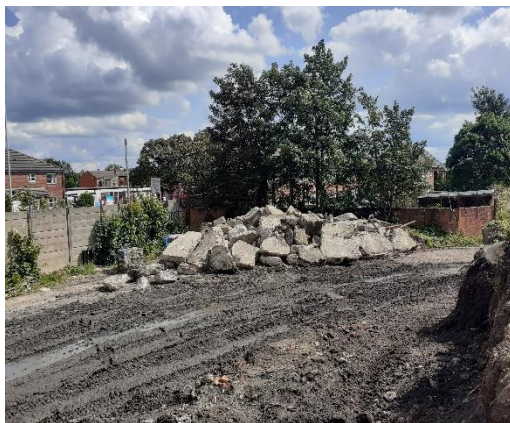
Photo 35: Concrete pile after checking for JK
