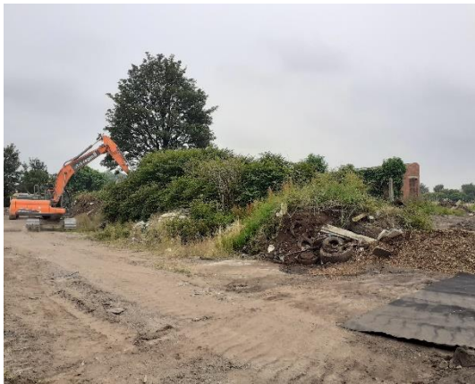
Photo 21: Japanese Knotweed banking before excavating
