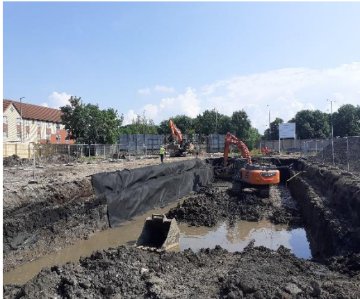
Photo 31: Burial cell 2 with cutex lining being done
