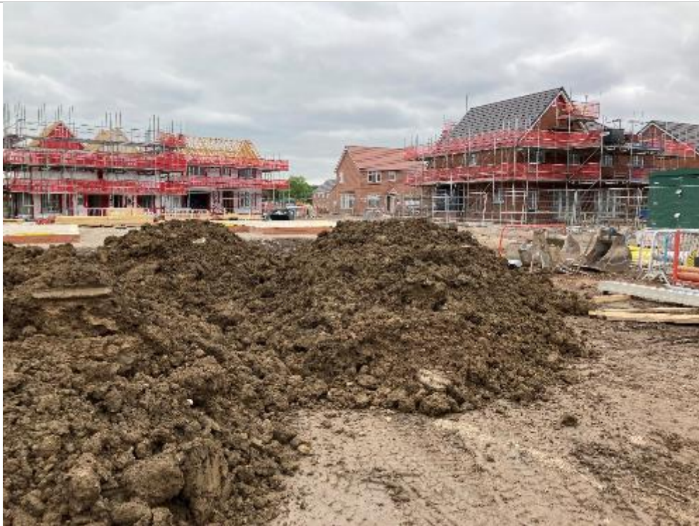
PLATE 32 SITE CLEARANCE- MADE GROUND TURNED IN THE WEST
