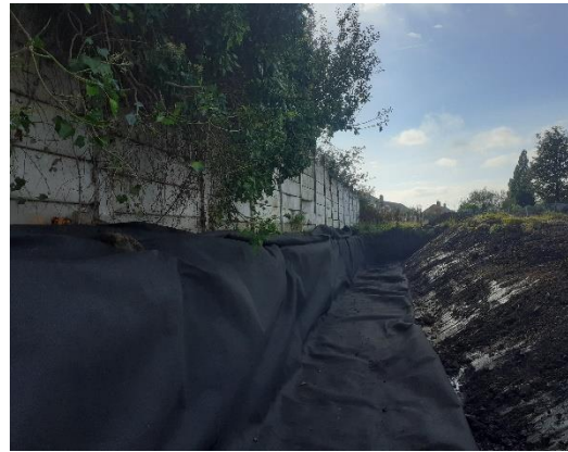
Photo 10: Japanese Knotweed area 3-4 with cutex before backfilling
