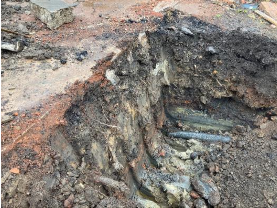
PLATE 23 CHEMICAL VALIDATION OF ELECTRICAL SUBSTATION
