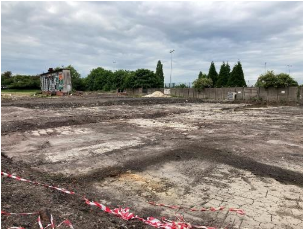
PLATE 6 SITE CLEARANCE- MADE GROUND TURNED IN THE WEST
