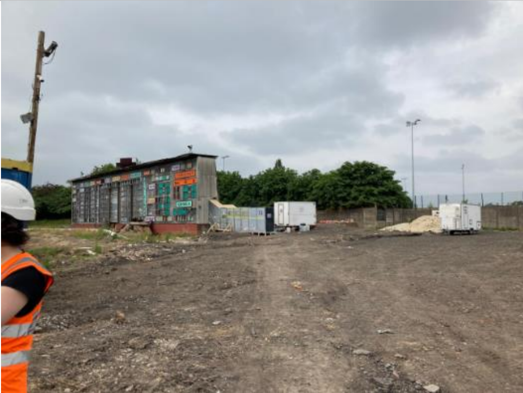
PLATE 15 ASBESTOS REMOVAL FROM THE SCOREBOARD
