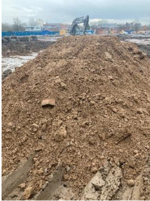
PLATE 31 IMPORTATION OF GRANULAR BULK FILL
