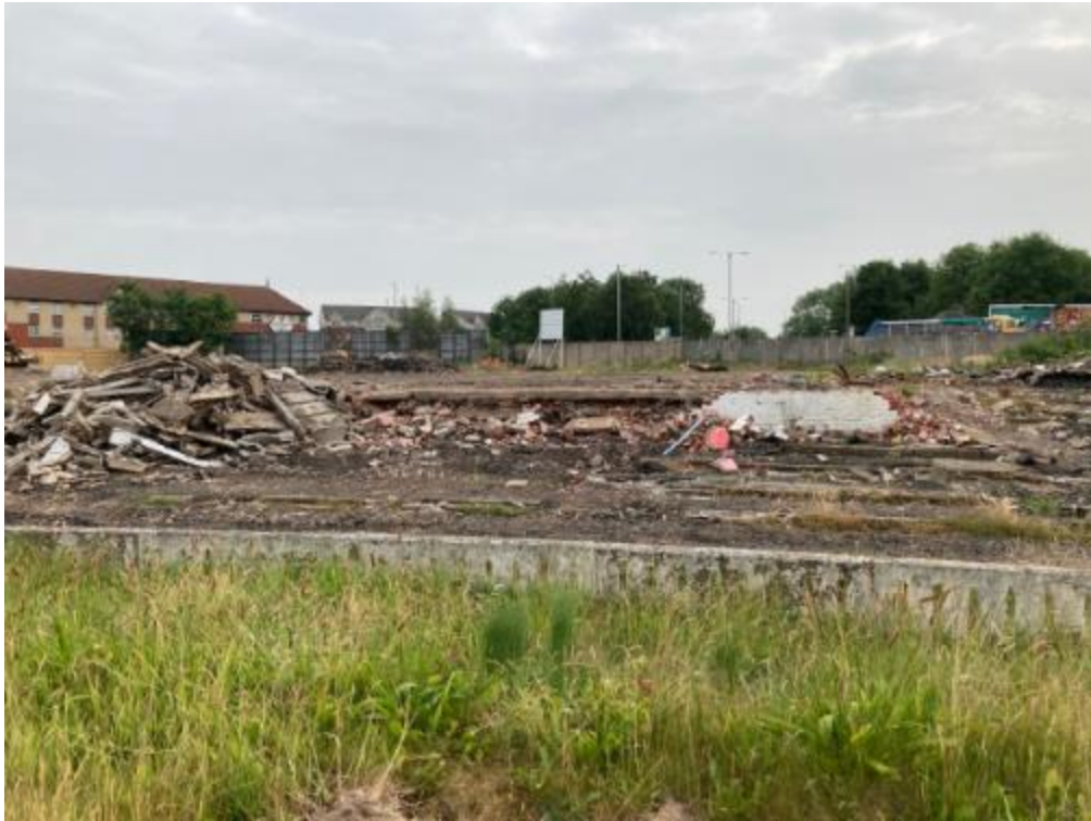
PLATE 9 SITE CLEARANCE – DEMOLITION OF STRUCTURES
