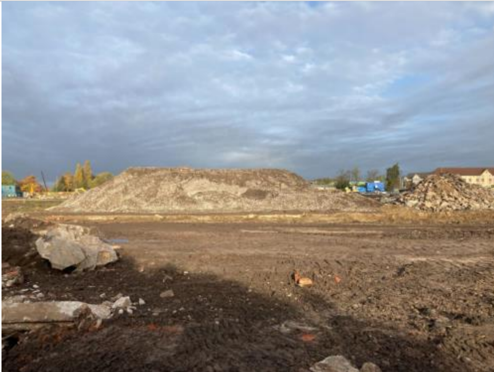
PROCESSING OF SUBSTRUCTURES AND MADE GROUND
