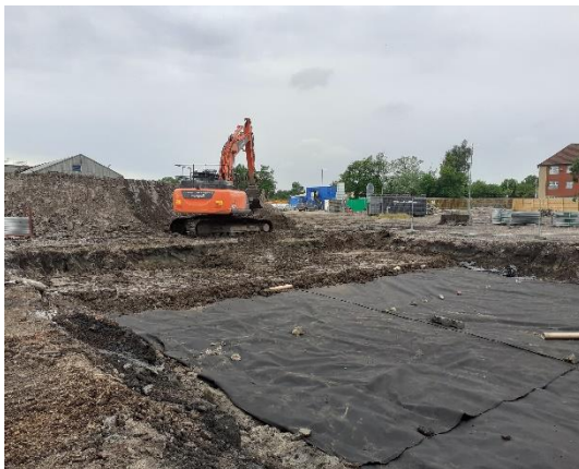
Photo 27: Burial cell No1 being backfilled with clean material
