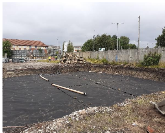
Photo 30: Burial cell No1 covered in cutex
