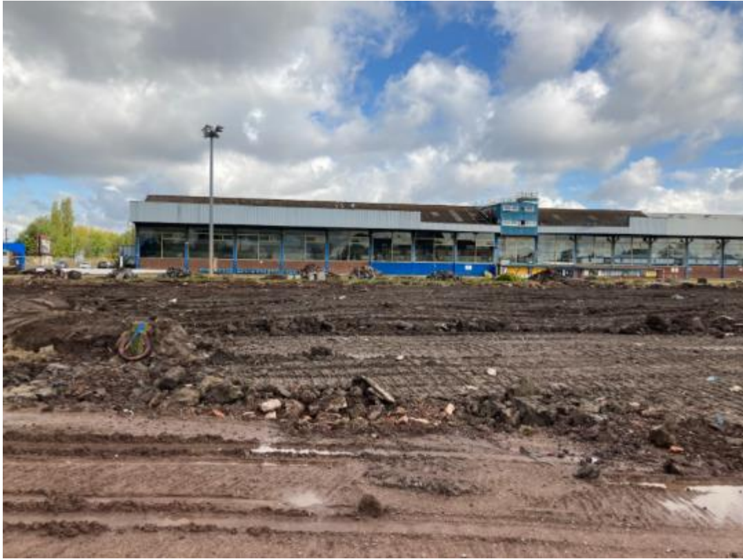
PLATE 5 MADE GROUND TURNED IN THE CENTRE OF SITE MAY 2021
