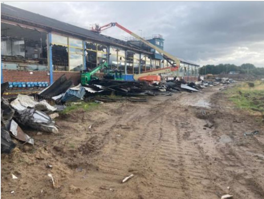
PLATE 14 ASBESTOS REMOVAL IN BULIDINGS
