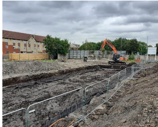
Photo 32: Burial cell 2 filled with JK impacted soil ready for top covering of cutex
