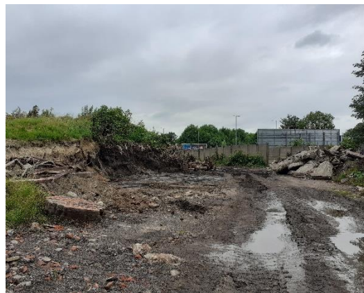
Photo 36: Farthest edge of banking area complete
