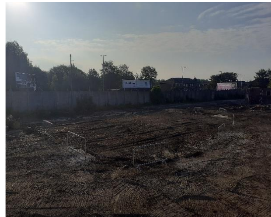
Photo 28: Burial cell No1 fully covered with clean material
