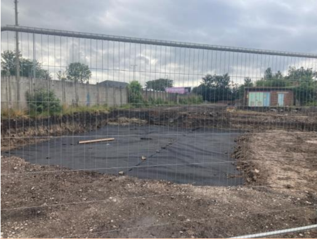
PLATE 13 JAPANESE KNOTWEED CELL IN THE EAST OF THE SITE
