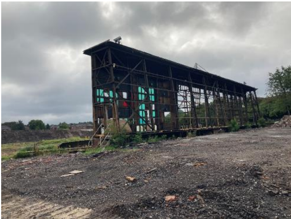
PLATE 8 SITE CLEARANCE- DEMOLITION OF STRUCTURES
