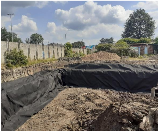
Photo 25: Burial cell 1 with cutex along edges
