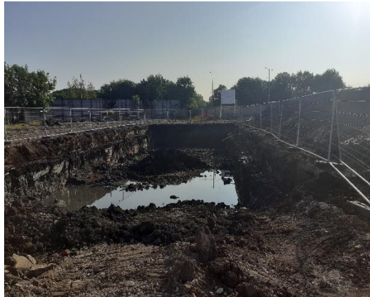
Photo 26: Burial cell No1 before backfilling
