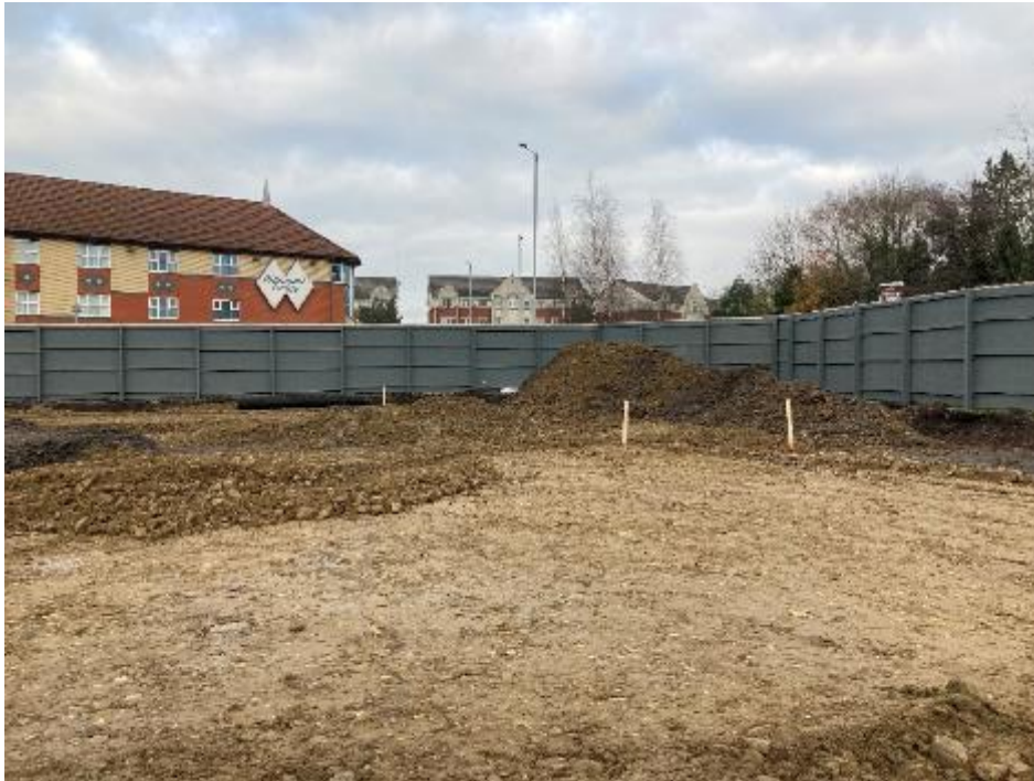
SITE CLEARANCE- MADE GROUND TURNED IN THE WEST
