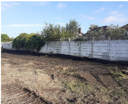
Photo 11: Japanese Knotweed area 3-4 with CuTex complete
