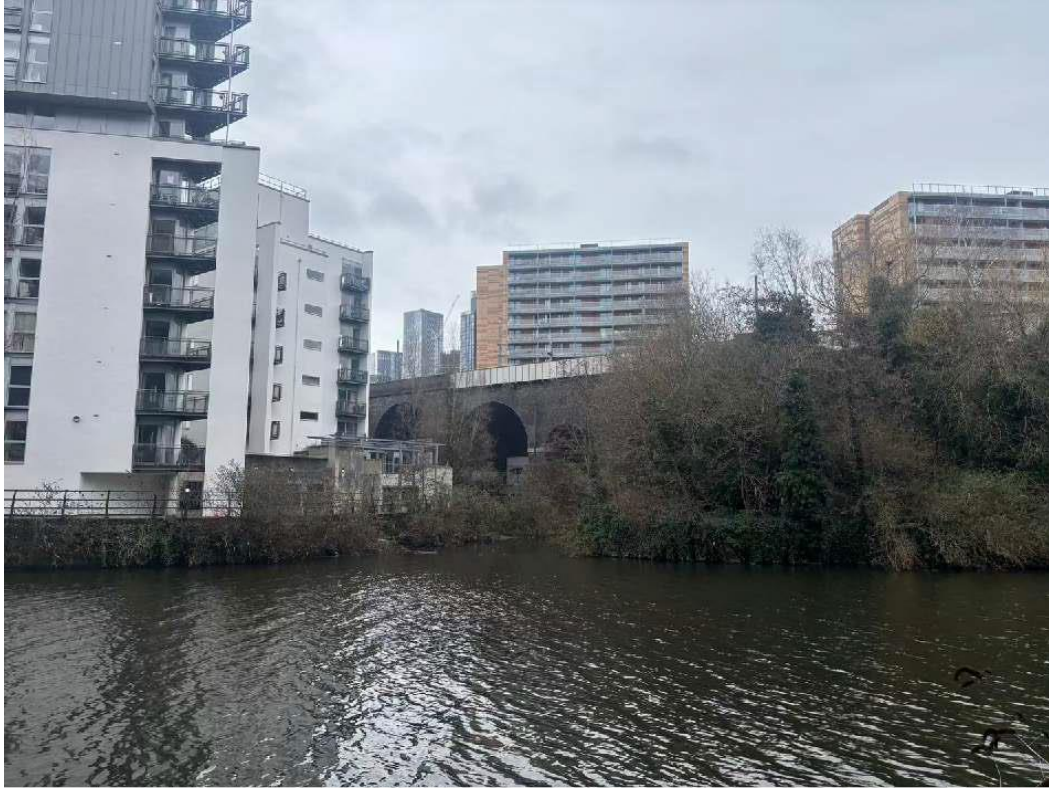
Figure 3: Looking southeast from the western towpath of the River Irwell, from next to the Riverside building.
