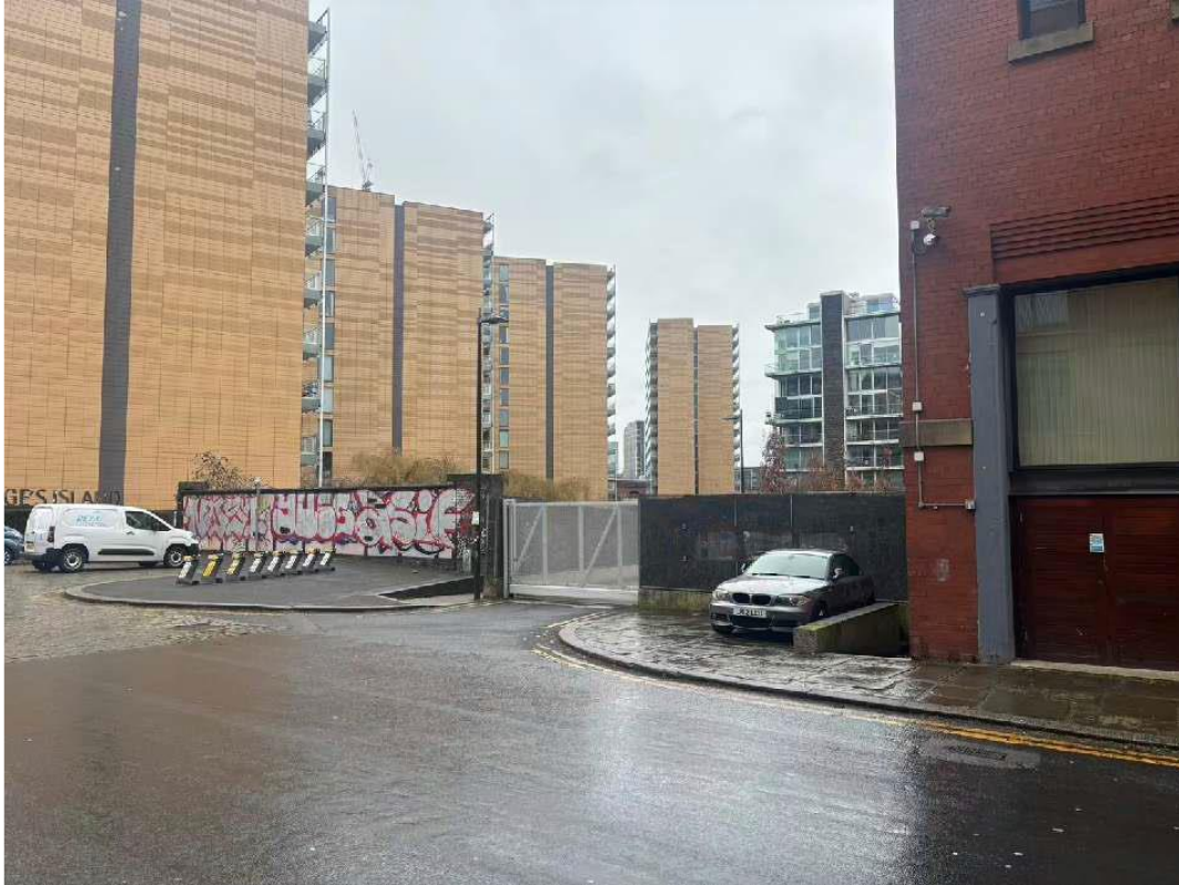
Figure 1: Looking north east from Hulme Hall Road.
