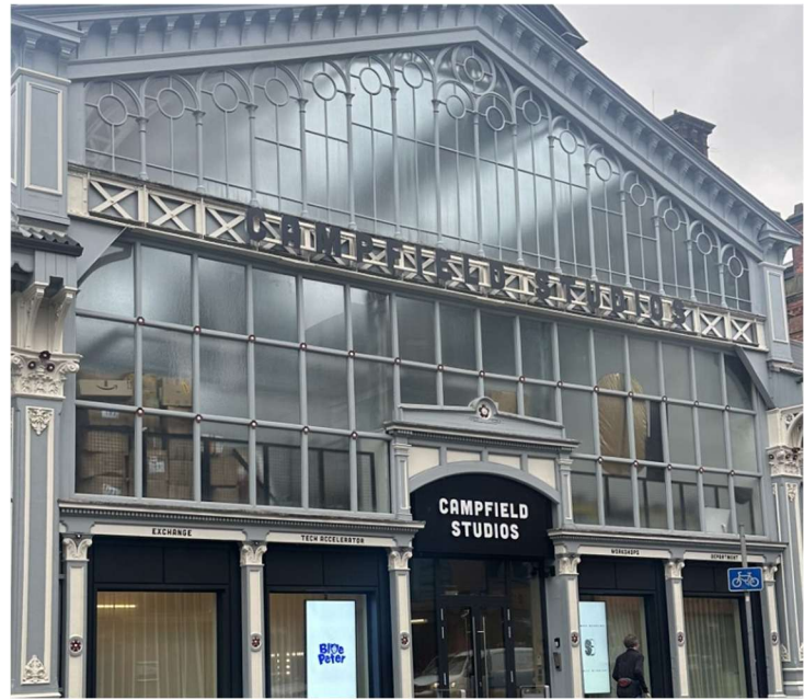
Permanent fascia, temporary vinyl and above door signage at Liverpool Road.
