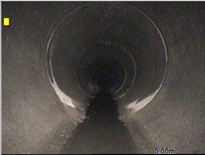
Start node type, manhole, reference S44
