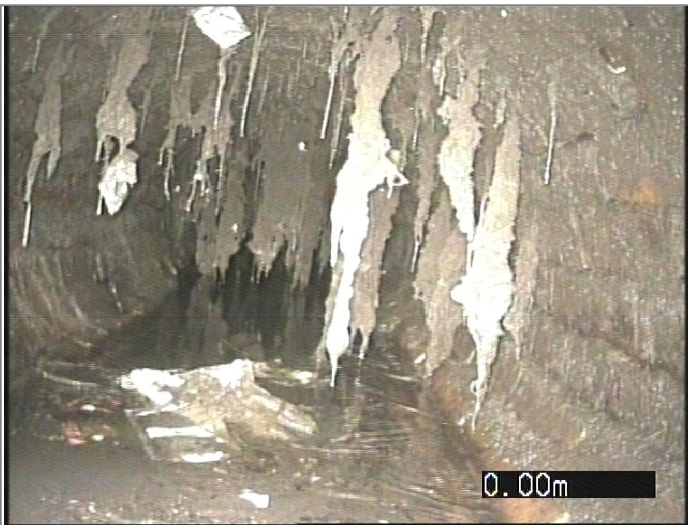
Start node type, manhole, reference UCMH01
