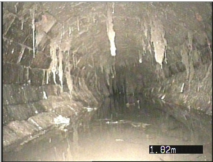
Start node type, manhole, reference UCMH01
