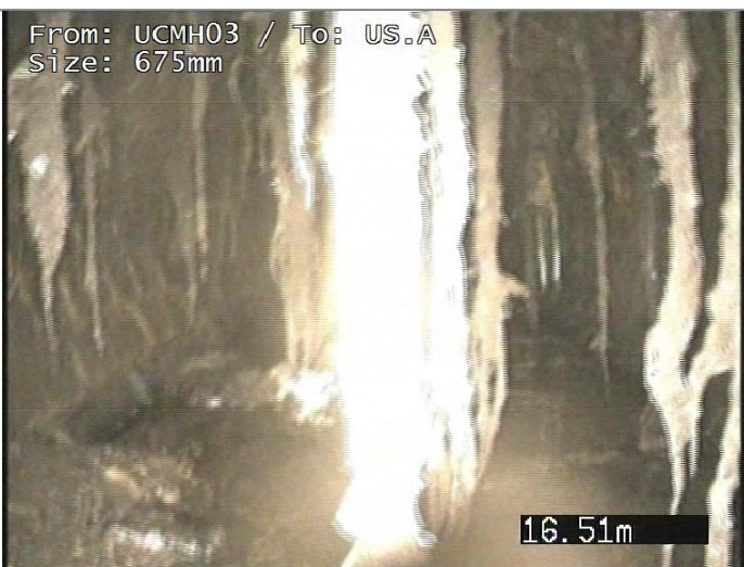
- Roots mass 25% cross-sectional area loss, Changed
