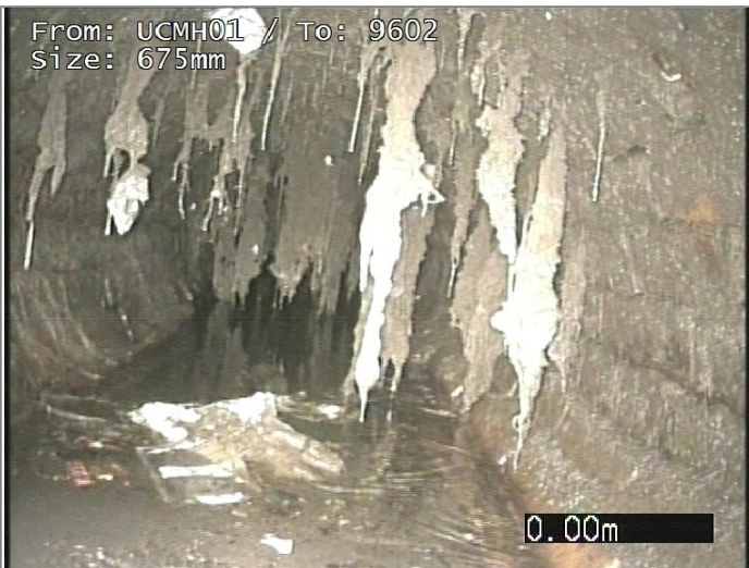
- Roots mass 30% cross-sectional area loss, Changed
