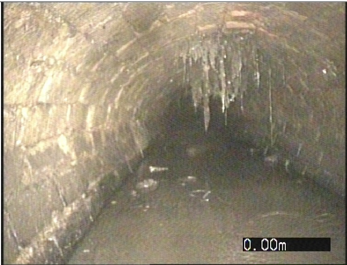
Start node type, manhole, reference UCMH03
