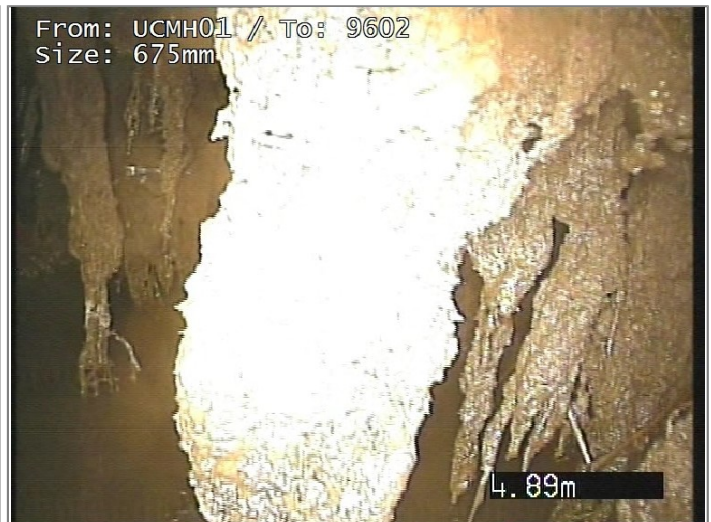
- Roots mass 50% cross-sectional area loss, Changed
