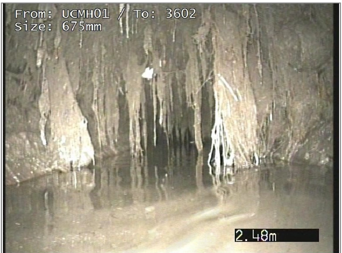
Roots mass 30% cross-sectional area loss, Changed
