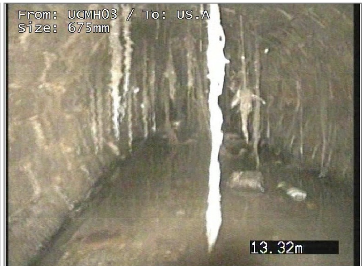
- Roots mass 10% cross-sectional area loss, Changed
