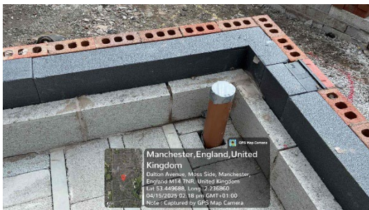
1C (E5) - Plot 5 - BEWI external perimeter wall
