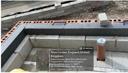
1C (E5) - Plot 5 - BEWI external perimeter wall
