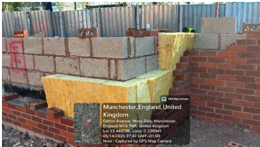
2A (E5) - Plot 5 - wall insulation above the cavity tray
