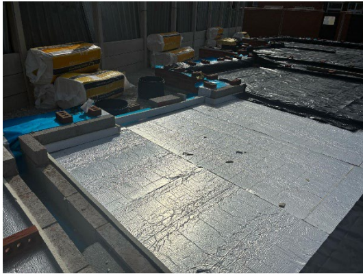
1A and 1C (E5) - plot 5 - floor screed GF perimeter insulation
