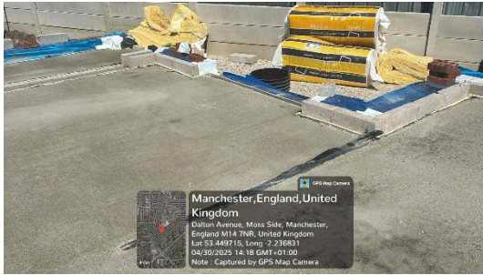
1A (E5) - plot 5 - Screed and perimeter insulation
