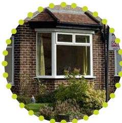
Dark red/ brownish brickwork to front
