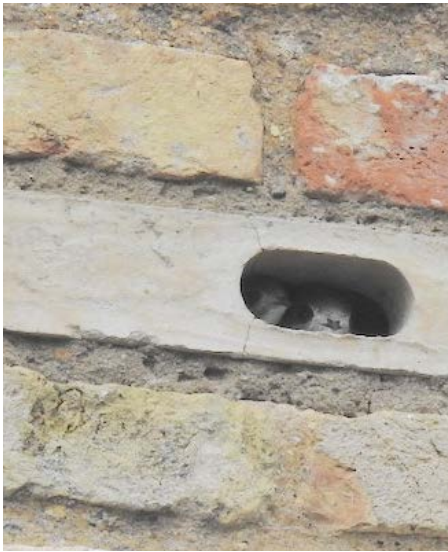
Swift Bricks- Side Elevation
