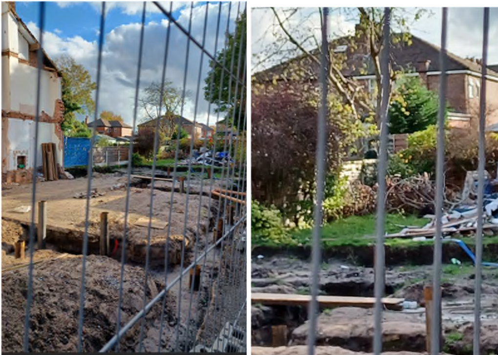
Views of the site facing east
