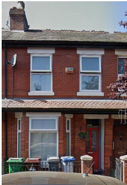
The application site
