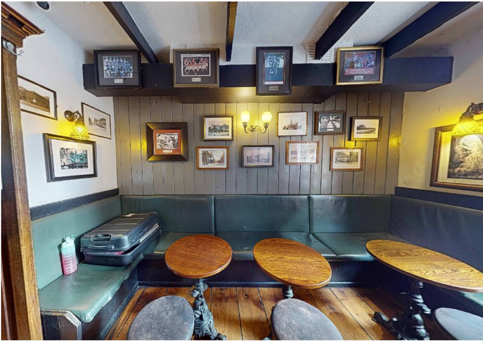
Existing Photo - Interior - Existing panelling and Fixed Seating Panelling removed for strip out and replacement with new 144x14mm polished HW reed and bead vertical panelling. Fixed Seating proposed for reupholstery Timber floor proposed for light sanding and relacquer with new clear matt lacquer Walls and Ceiling proposed for decoration only Refer to:- DWG 3251 TGH 2.01C Proposed Ground Floor Plan - GA DWG 3251 TGH 2.02 Proposed Ground Floor Plan - Demolitions DWG 3251 TGH 2.03 - Proposed Ground Floor Plan - Builders Works
