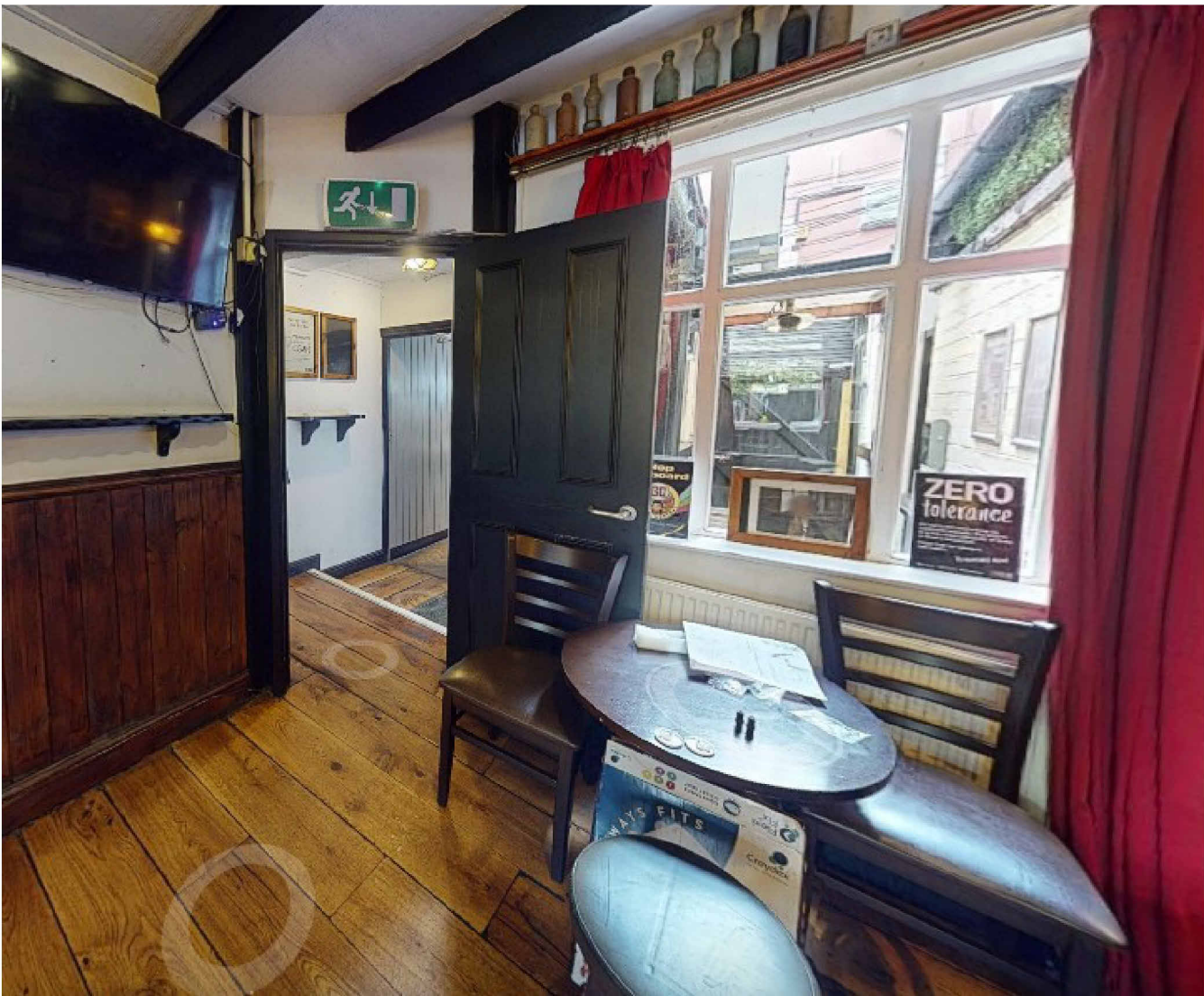
Existing Photo - Interior - Existing stud wall, door and rear window Proposed for removal including dropping of sill to floor level to create new door opening. Refer to:- DWG 3251 TGH 2.01C Proposed Ground Floor Plan - GA DWG 3251 TGH 2.02 Proposed Ground Floor Plan - Demolitions DWG 3251 TGH 2.03 - Proposed Ground Floor Plan - Builders Works
