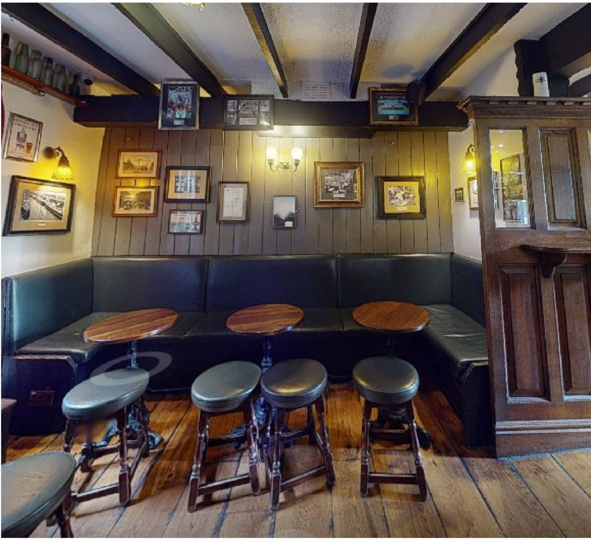
Existing Photo - Interior - Existing panelling and Fixed Seating Panelling removed for strip out and replacement with new 144x14mm polished HW reed and bead vertical panelling. Fixed Seating proposed for reupholstery Timber floor proposed for light sanding and relacquer with new clear matt lacquer Walls and Ceiling proposed for decoration only Refer to:- DWG 3251 TGH 2.01C Proposed Ground Floor Plan - GA DWG 3251 TGH 2.02 Proposed Ground Floor Plan - Demolitions DWG 3251 TGH 2.03 - Proposed Ground Floor Plan - Builders Works
