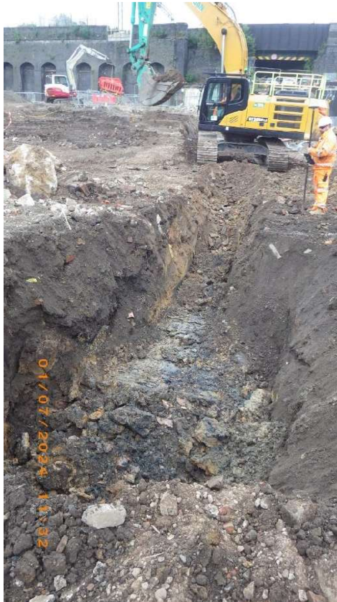
NT02 facing S. Removal of deeper drain runs
