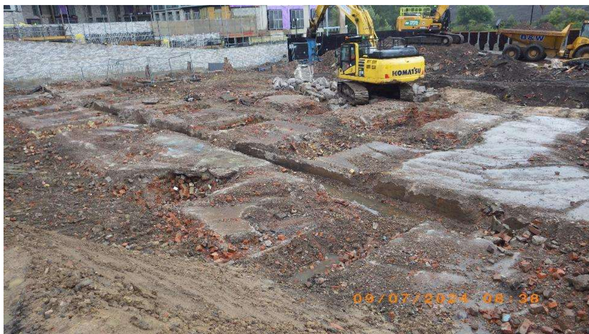
Further uncovering of buried obstructions, NT02 facing NW
