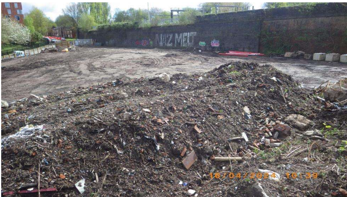
NT04: excavation of stockpiled knotweed material
