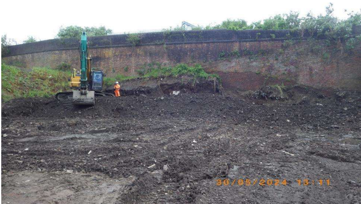
NT03 facing S towards viaduct: placement of materials for permanent upfill.
