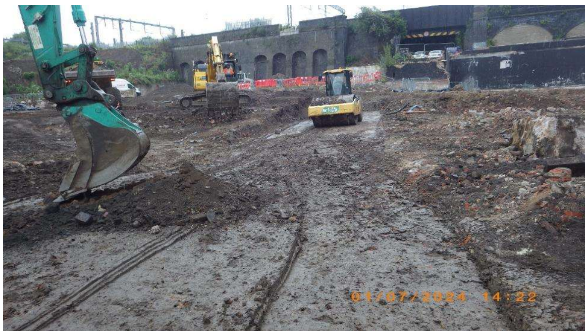
NT02: backfilling post drainage run chasing
