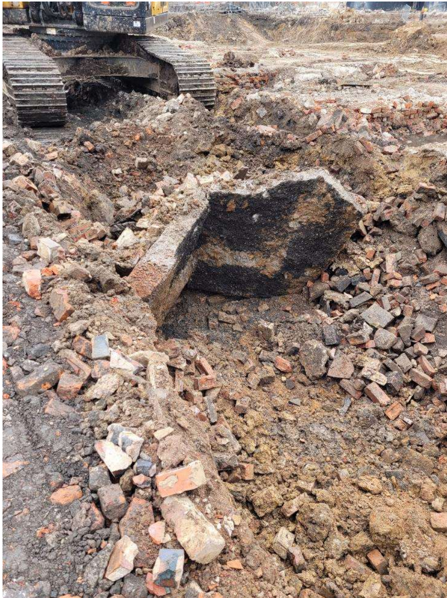
NT02: demolition of "NT02 tank"
