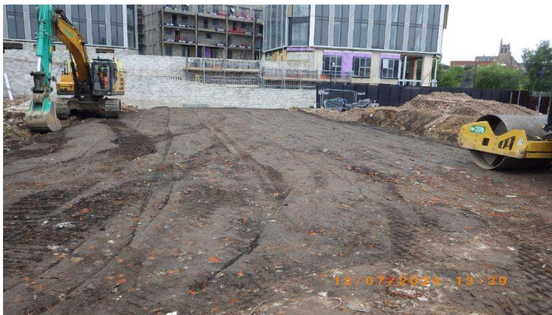
NT03: backfill and compaction following obstruction removal
