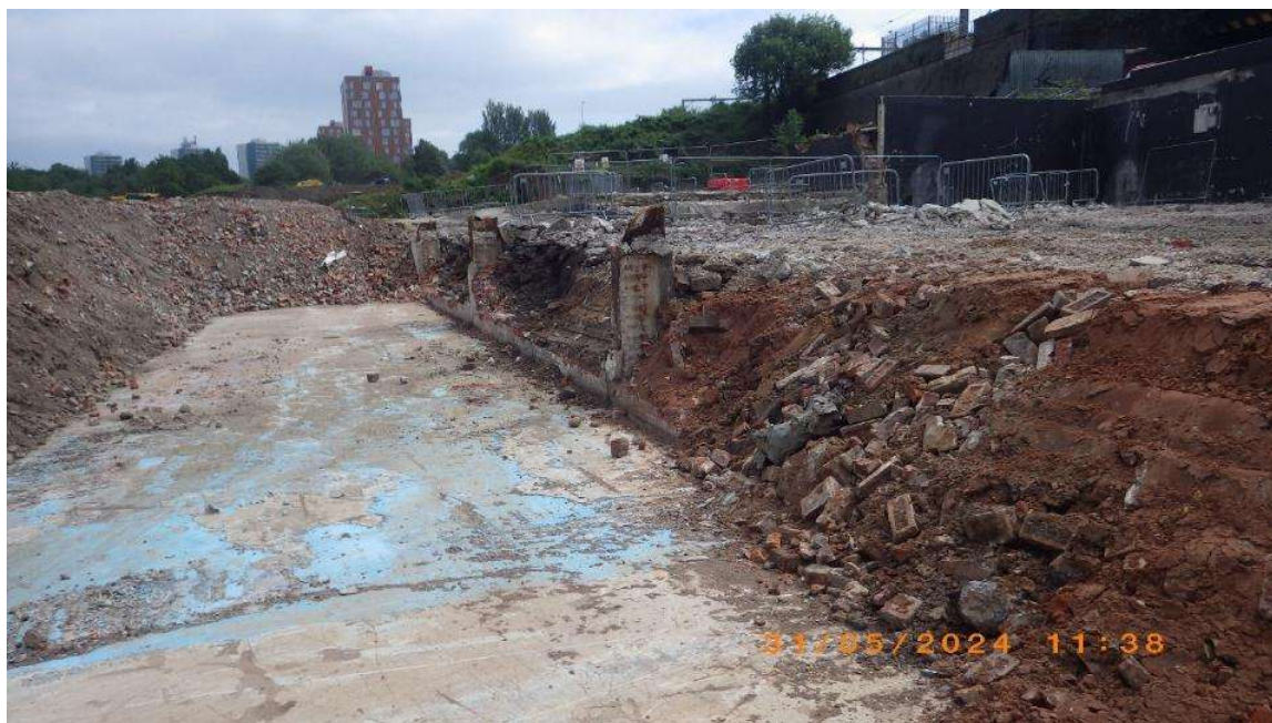
NT02 facing E: pre-excavation of TCE impacted materials. Note garage retaining wall to right 31 st May 2024
