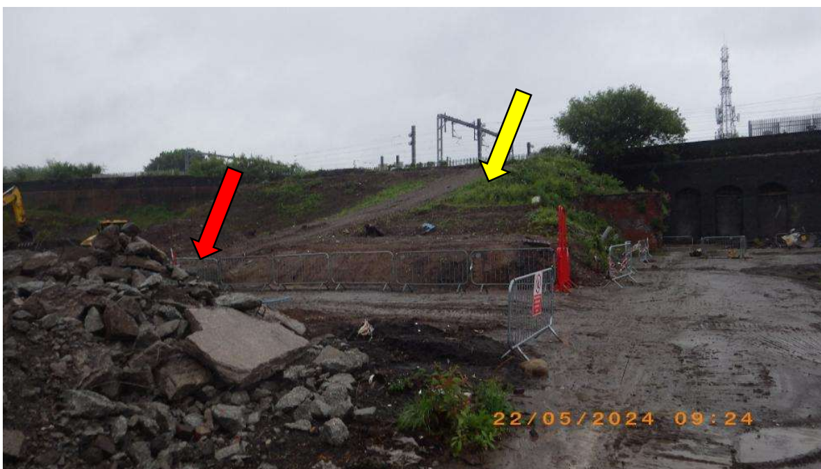
NT03 facing S towards railway viaduct. Note “ramp” (yellow arrow) and stockpiled oversized (red arrow)
