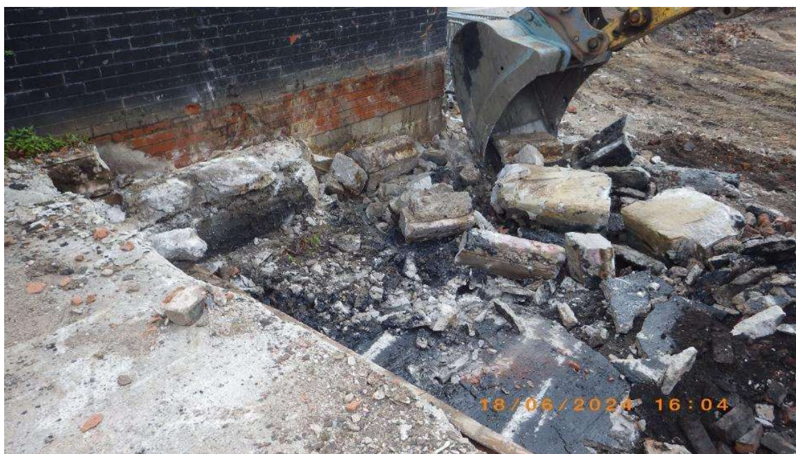
NT02/NT03: demolition of five chambered tank 18 th June 2024
