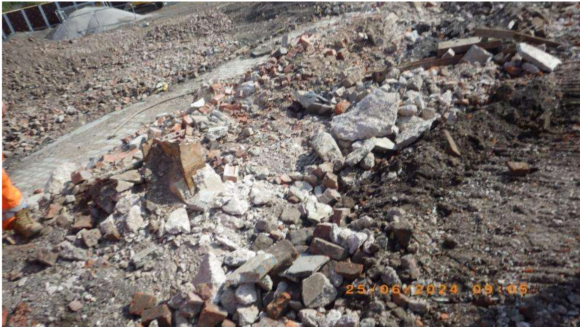
NT02: uncovering of obstructions (see Section 5)
