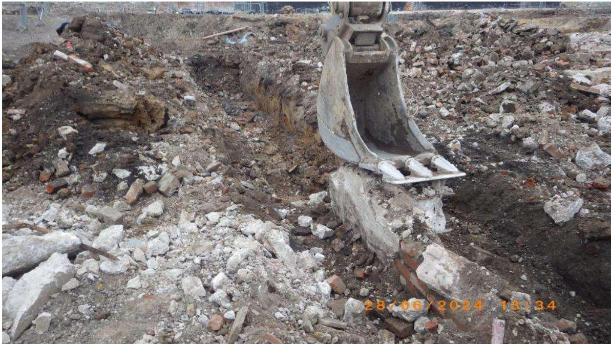
NT02, facing S. chasing of drainage runs
