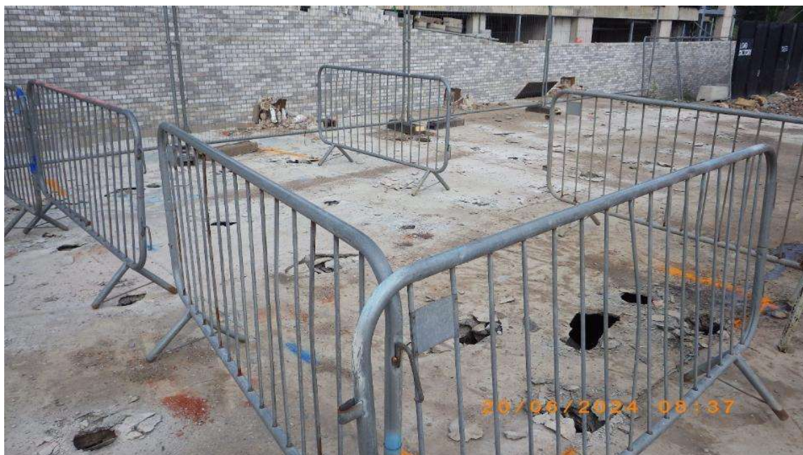
NT02 western boundary: "NT02 tank" encountered during demolition of floor slab (see Section 4.2)
