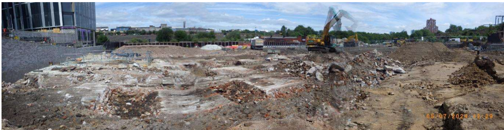
NT02 facing N from now-remediated TCE area. Note buried obstructions uncovered and about to be demolished
