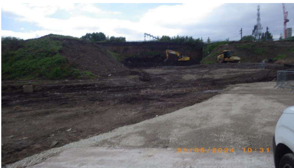
NT03 facing S: permanent upfill works
