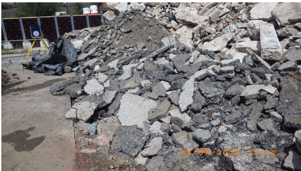
NT03 crushing area: segregation of tarmac to avoid contamination of 6F2.
