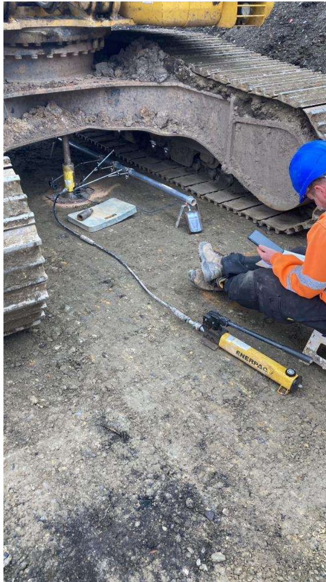
NT03 pile mat: final deformation plate tests
