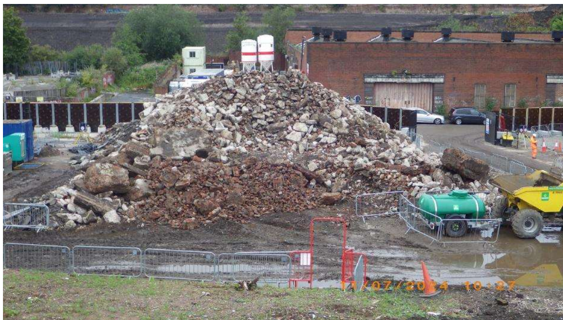
NT03: oversize stockpile awaiting arrival of crusher
