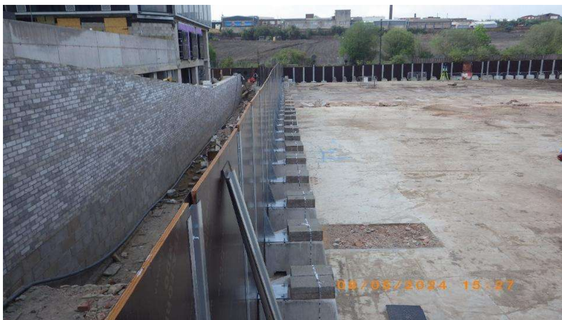
Western boundary of NT02, facing N. Boundary trench backfilled as part of works 8 th May 2024
