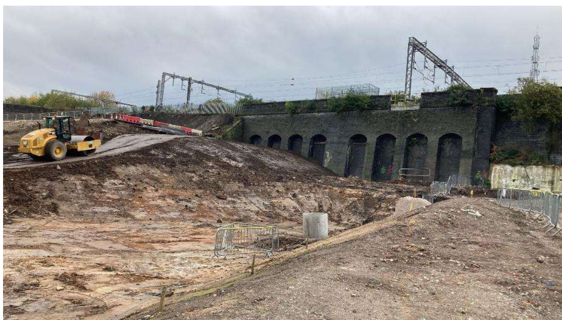
NT03 S boundary: extension of pile mat across area formerly occupied by MP gas main. Roller is compacting access road
