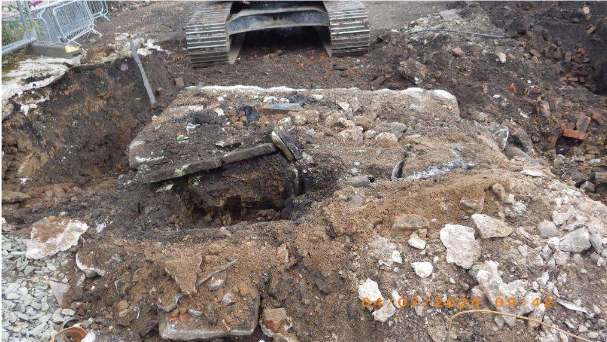
NT03 "small tank" demolition
