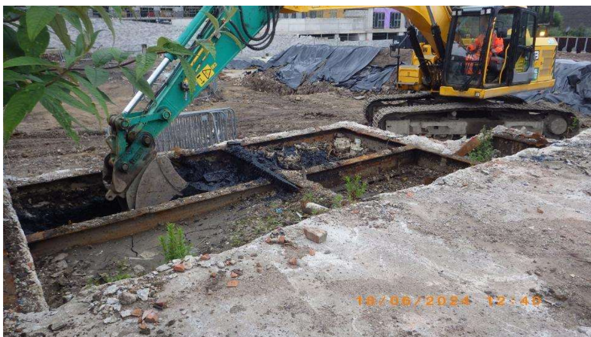
NT02/NT03: excavation of contents of five chambered tank (see Section 4.1)
