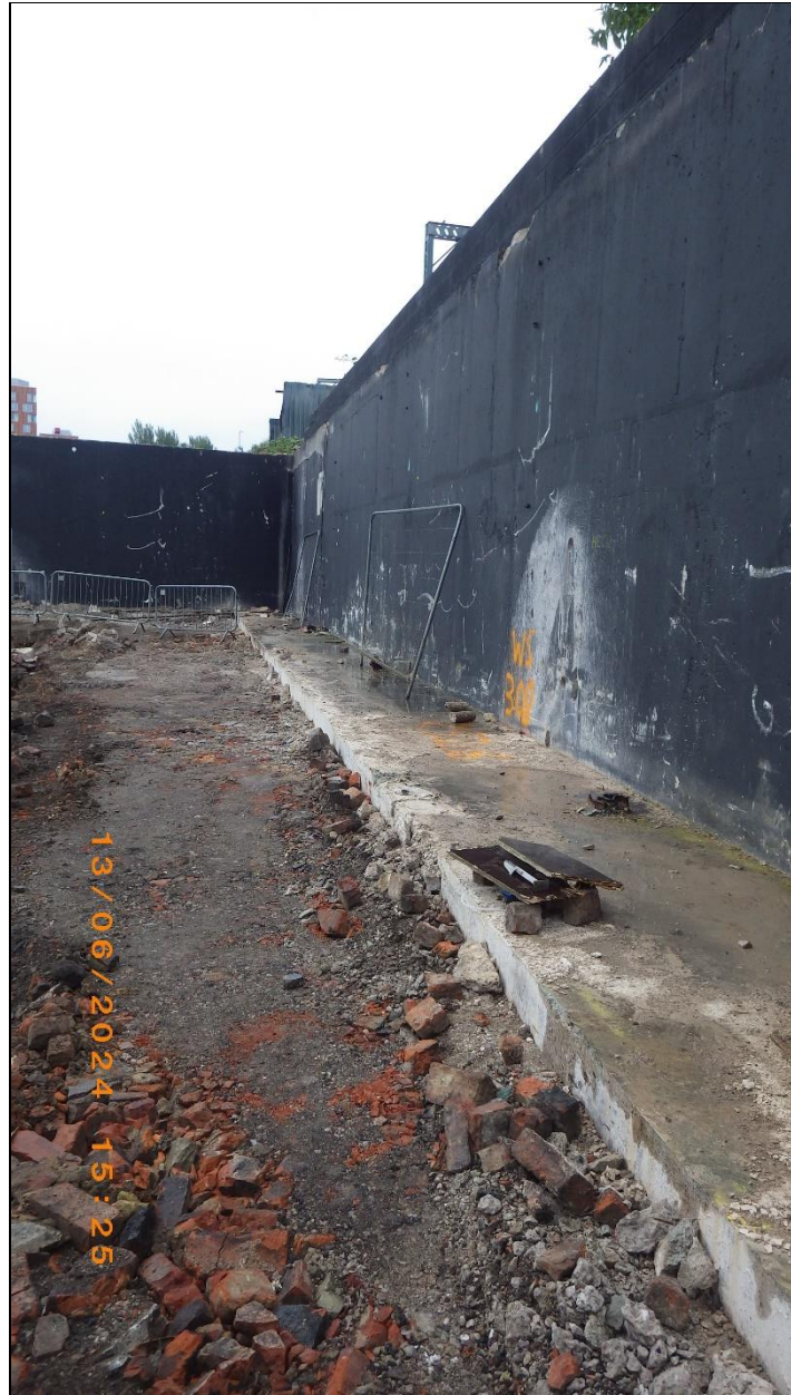
Facing east in TCE area. Note standoff from garage retaining wall to right
