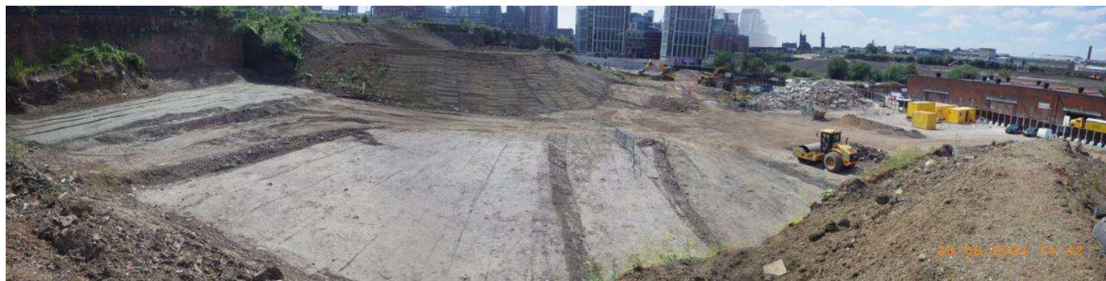
NT03 permanent uphill works, facing W (railway viaduct to left)
