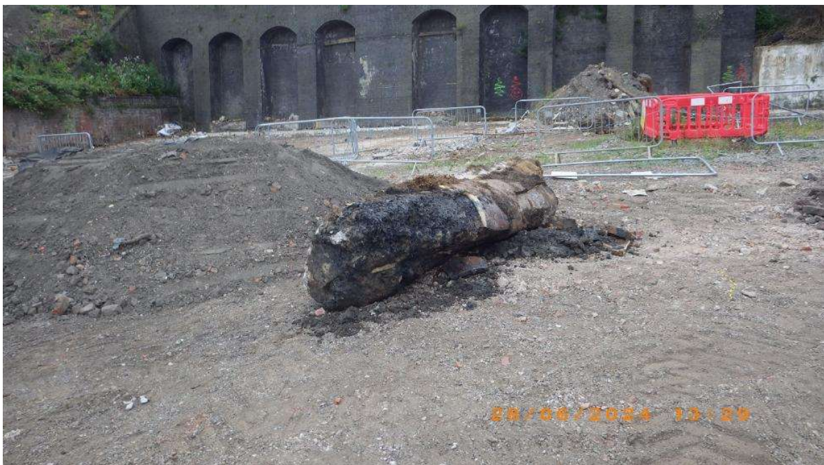
NT02: chasing and removal of drainage runs
