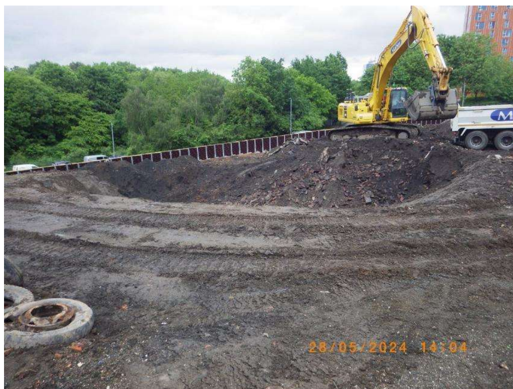
NT04 excavation and export works, as above
