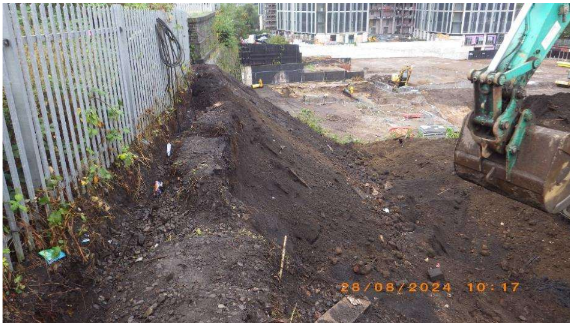
NT03, top of “ramp” on S boundary. Final cut. 28 th August 2024
