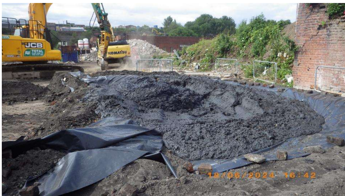
Contents of five chambered tank in sealed quarantine area 18 th June 2024
