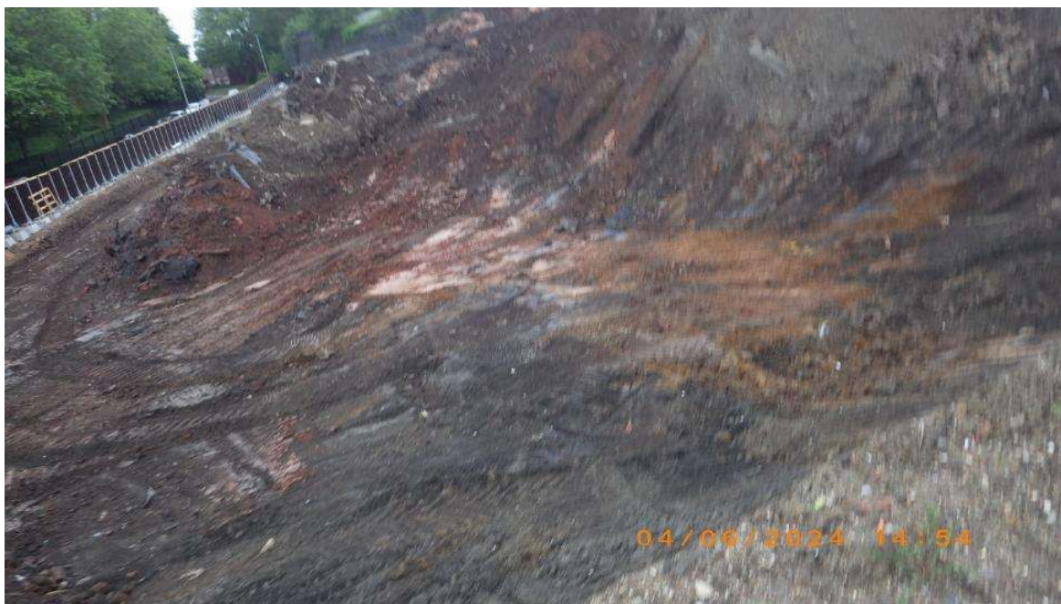
NT04 facing E. excavation & export cont'
