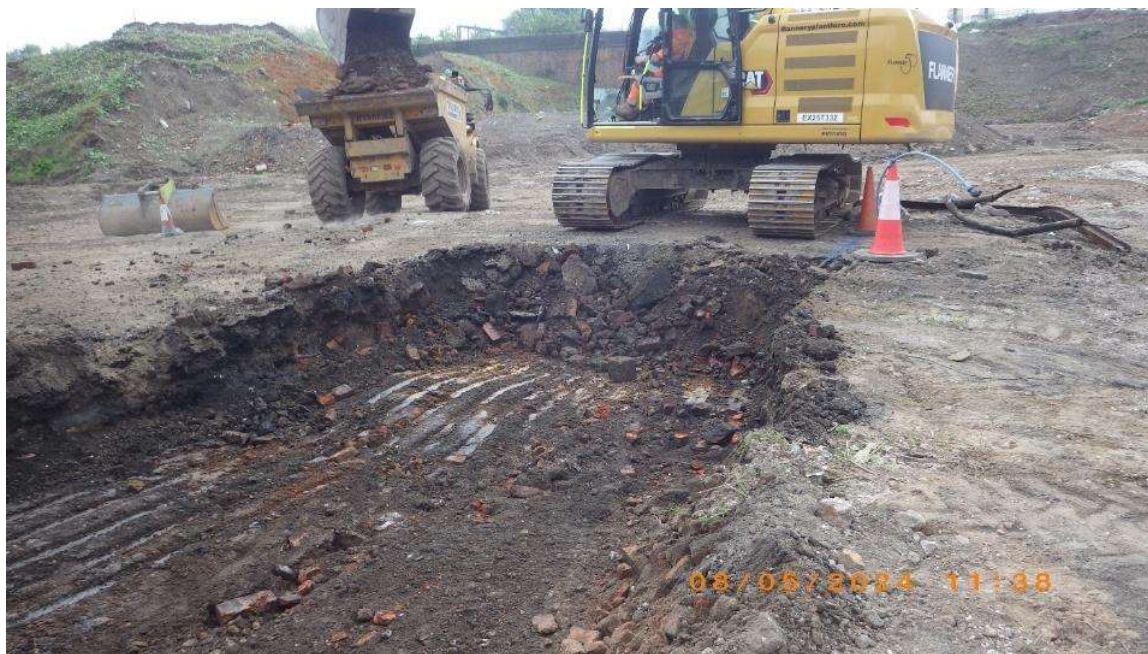
NT03 facing S: clearance works for site compound. Note small quantity of asbestos cement encountered within fill materials in this location: removed to quarantine area (see page 6)
