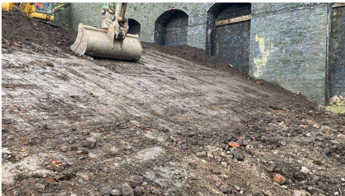
NT03 S boundary: shaping of batter on extension of pile mat across area formerly occupied by MP gas main
