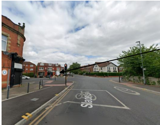
View north along Slade Lane as existing.
