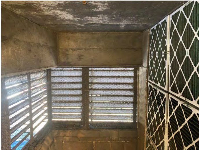
Photograph 13: Air con unit attached to 7th floor plant room
