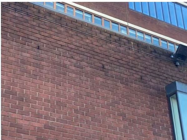
Photograph 3 : Weep holes present on the exterior of MMU library building (B01)
