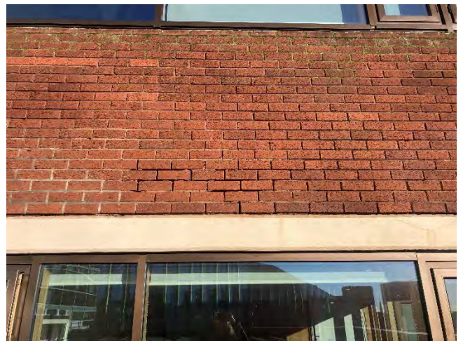
Photograph 18 and 19: Level 3 flat roof with solar panels and gaps in mortar present in brickwork
