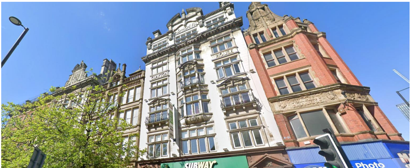
Piccadilly elevation of Grade II listed Gardens Hotel and shops (51-57 (odd) Piccadilly, Manchester, M1 2AP), Clayton House, 59, Piccadilly and 61 Piccadilly, and St Margarets Chambers
