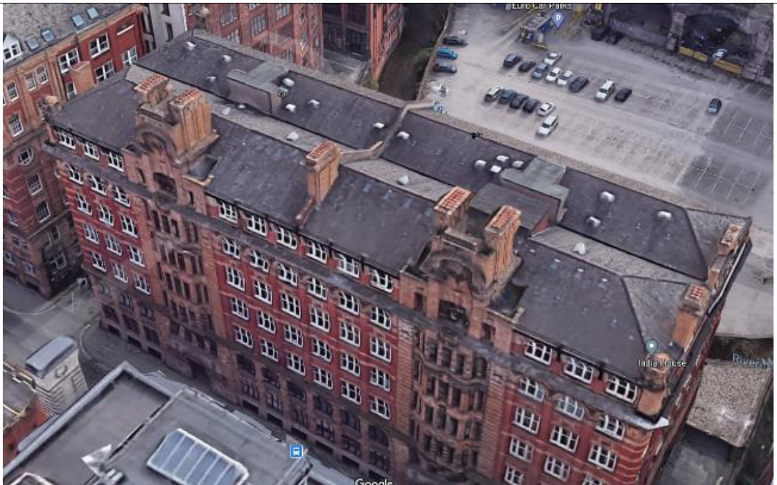
North (Front) Roof
