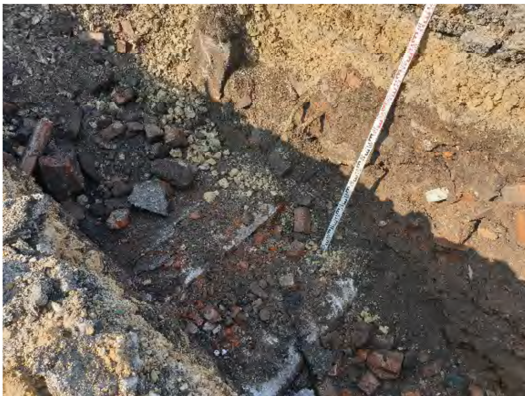
Photo No. 5: TPI03
