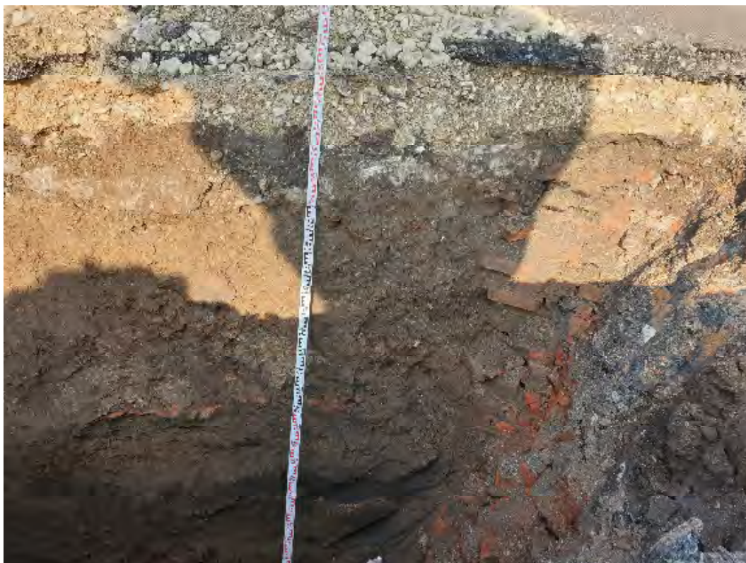
Photo No. 7: TPI04
