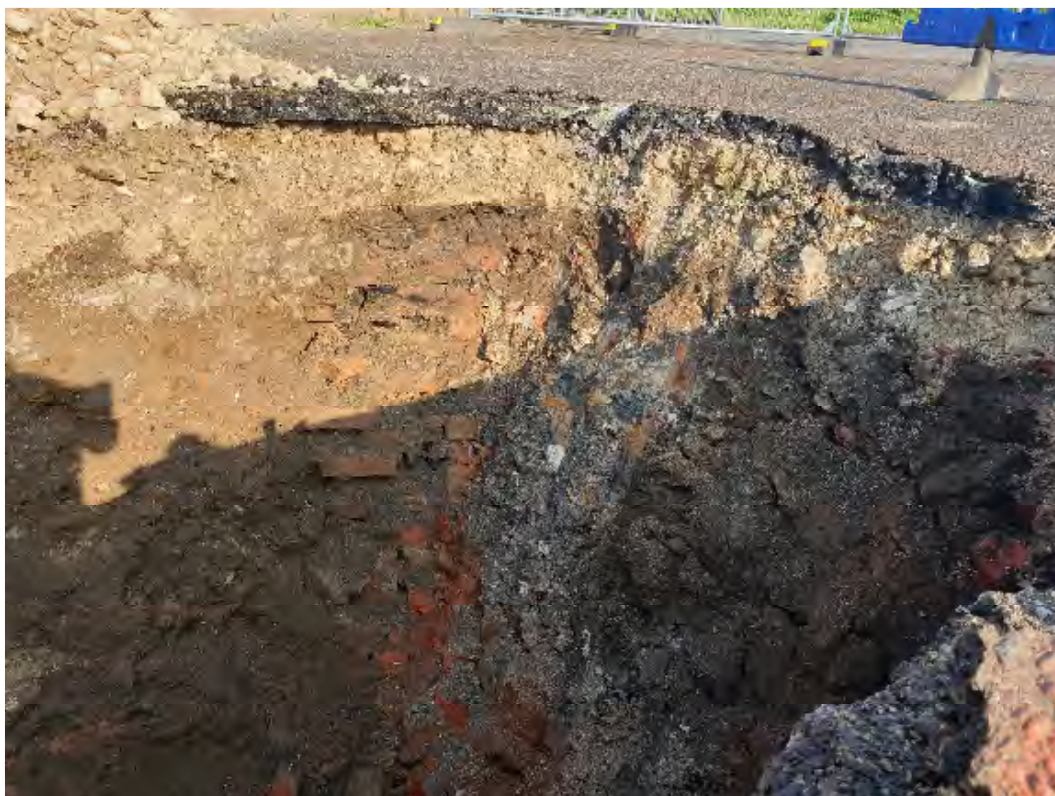
Photo No. 8: TPI04
