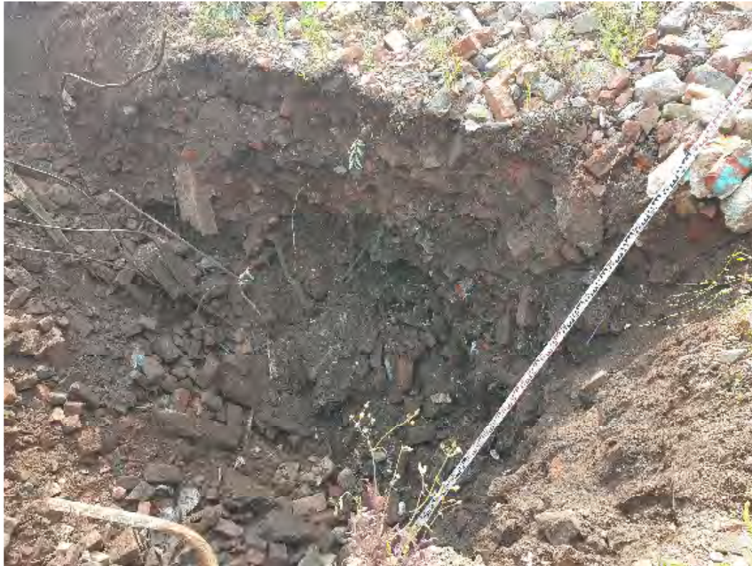
Photo No. 1: TPI01
