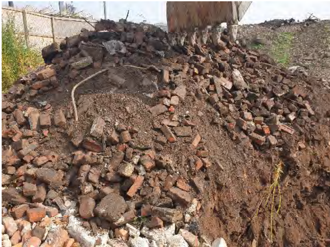
Photo No. 2: TPI01 Arisings
