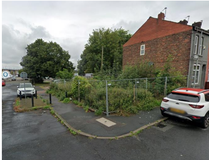
Figure 1 Street view of site
