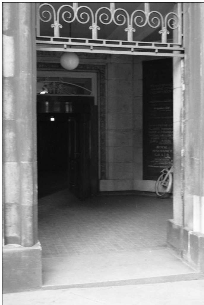
Figure 23 - Photograph dating to 1958, showing the original lobby.
