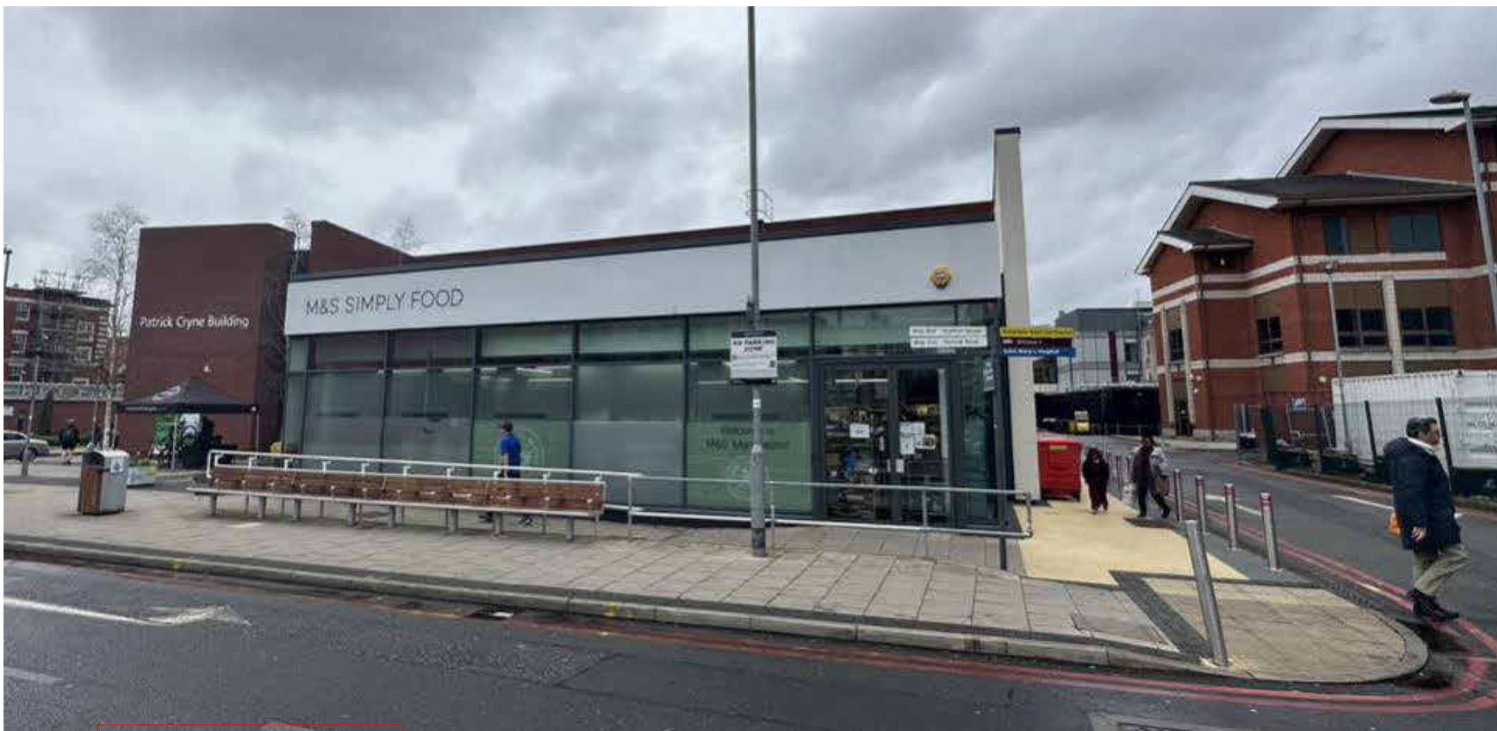
EXISTING ELEVATION PHOTO 2
