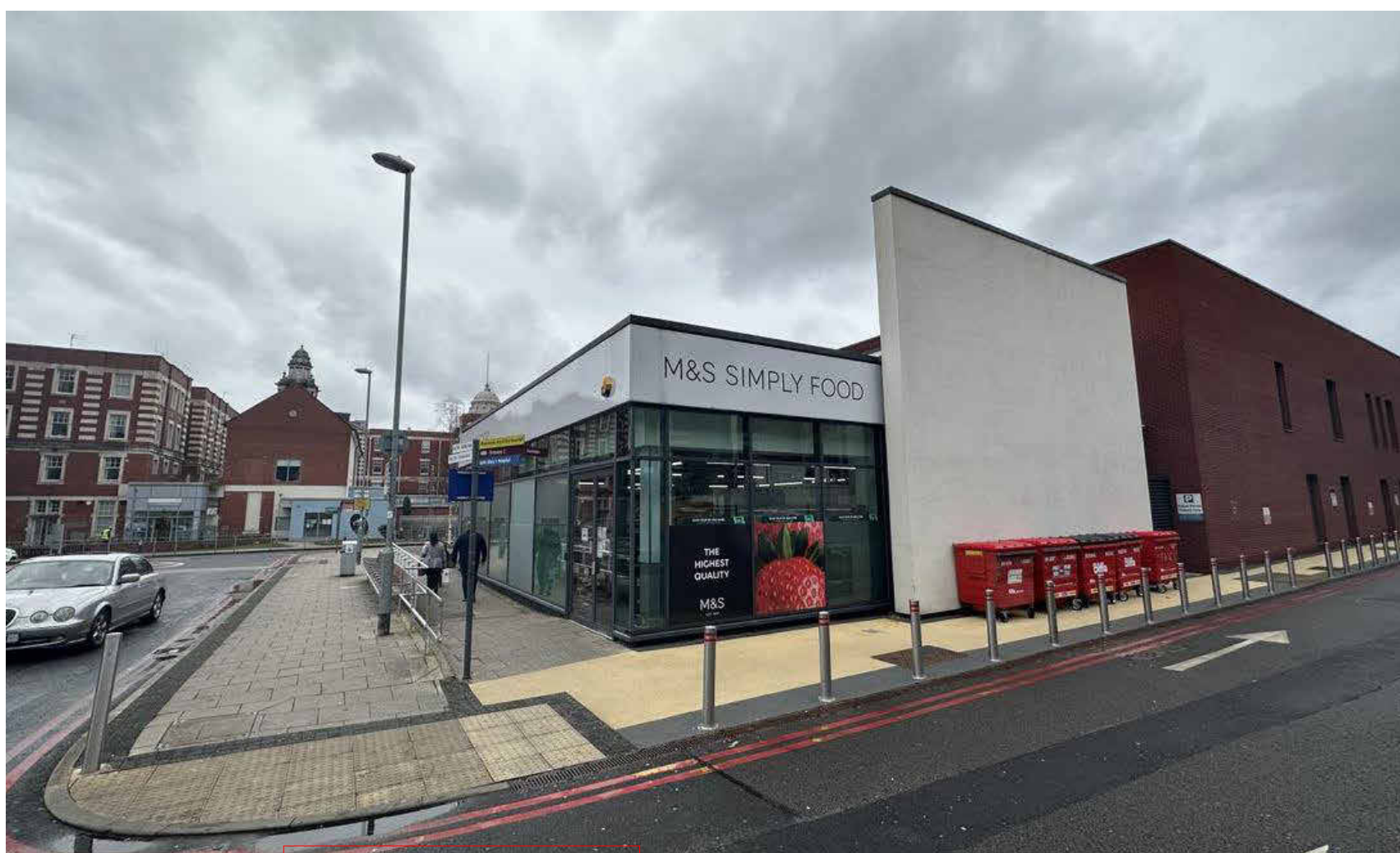
EXISTING ELEVATION PHOTO 3
