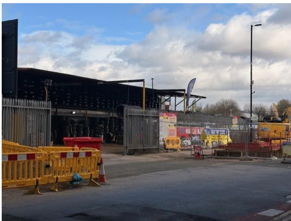
View from Fairfield Street
