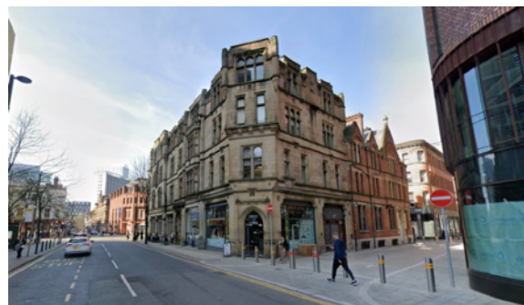
View of Building from John Dalton Street looking down Ridgeway
