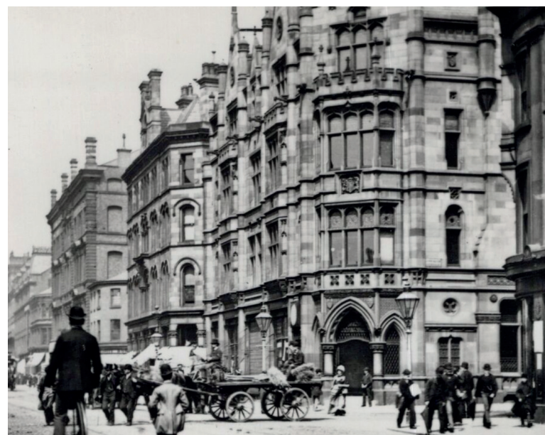
Image 6: Historic photograph of building, as viewed from Deansgate in late 19th century.
