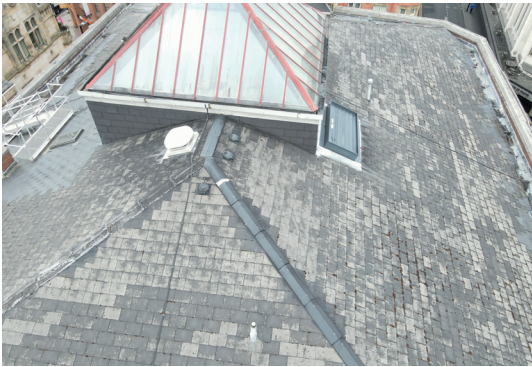
Image 15: Wider context of lantern position on roof, taken before current works commenced.
