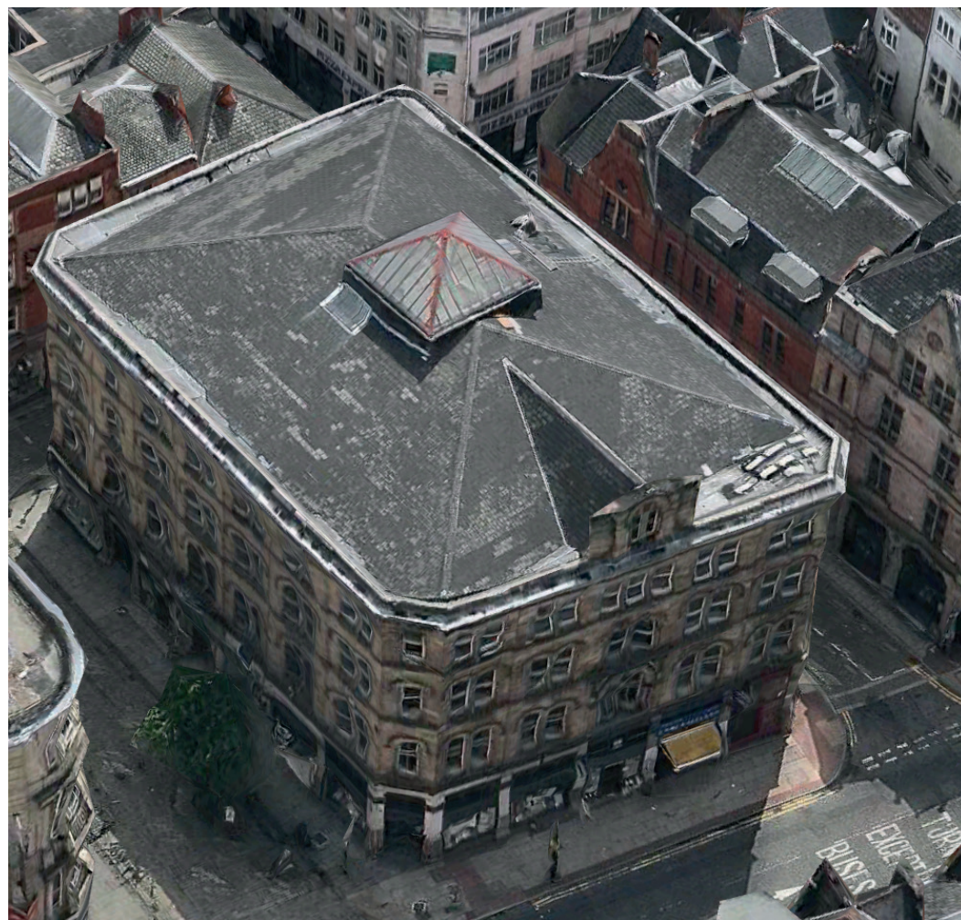
Image 2: Aerial image of the property showing the altered roof with central pyramid roof light, before recent works commenced.
