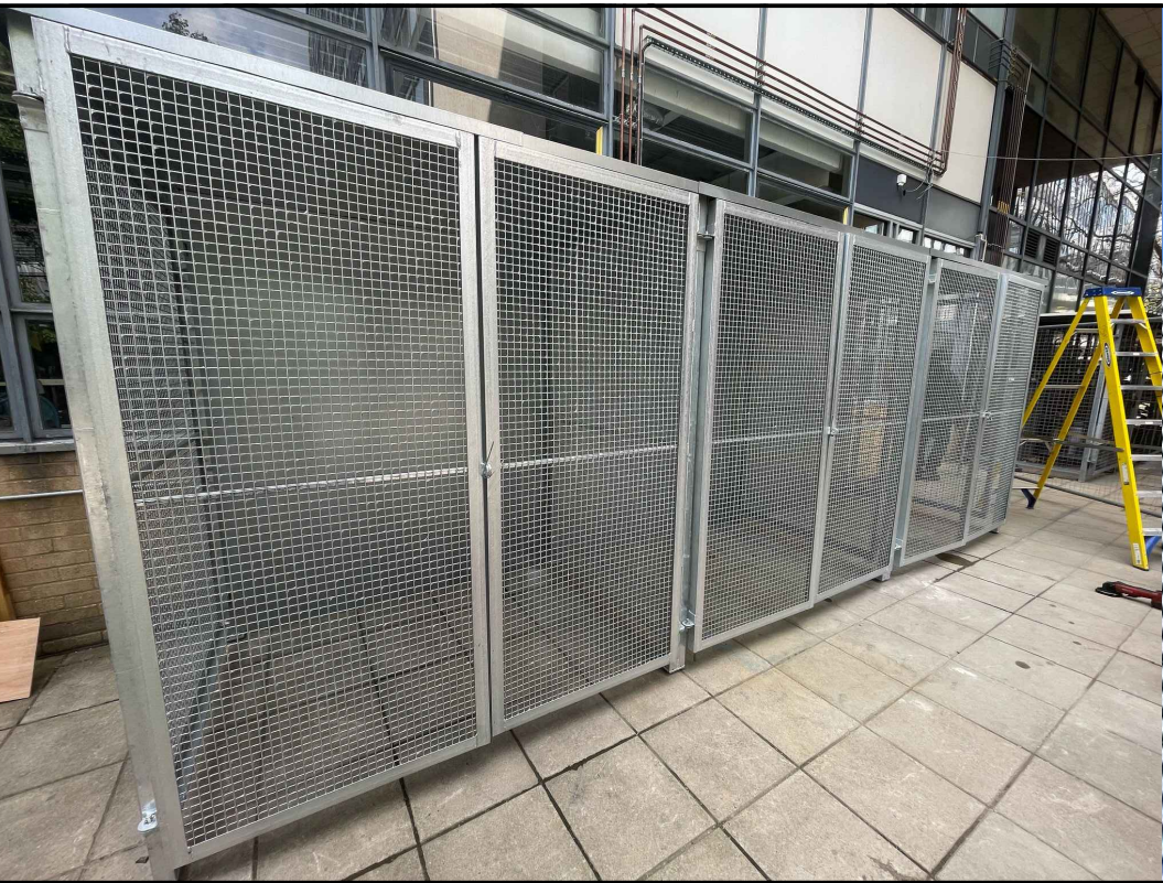
PROPOSED MESH SCREENS AND FRAMES FOR BOTTLES STORE Steel mesh and frames to match existing formats Moncaster Wire Products in galvanised grey finished
