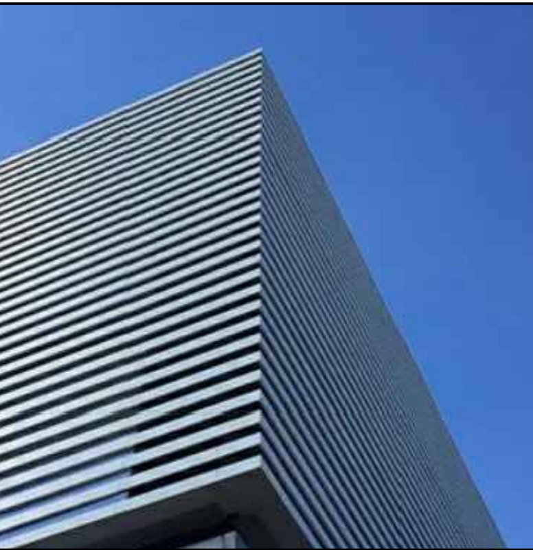
PROPOSED LOUVRES FOR PLANT ROOM Aluminium profiles steel frames concealed behind Caïse SS300 'Continuous Line' in mid-grey RAL7012
