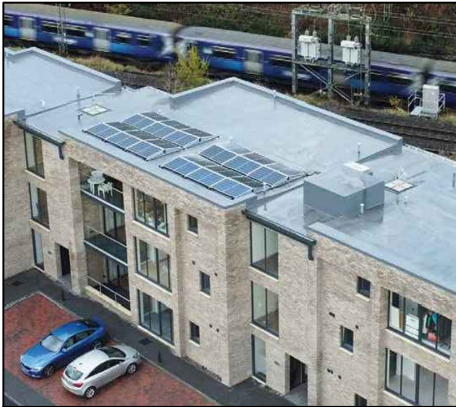
PROPOSED PLANT ROOM & CANOPY ROOF Single ply membrane IKO Armourplan P in mid-grey finish: Colour RAL7046
