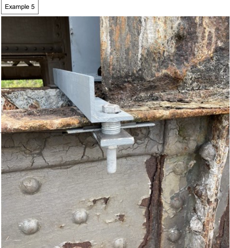
Washers as packers across top flange of bottom chord
