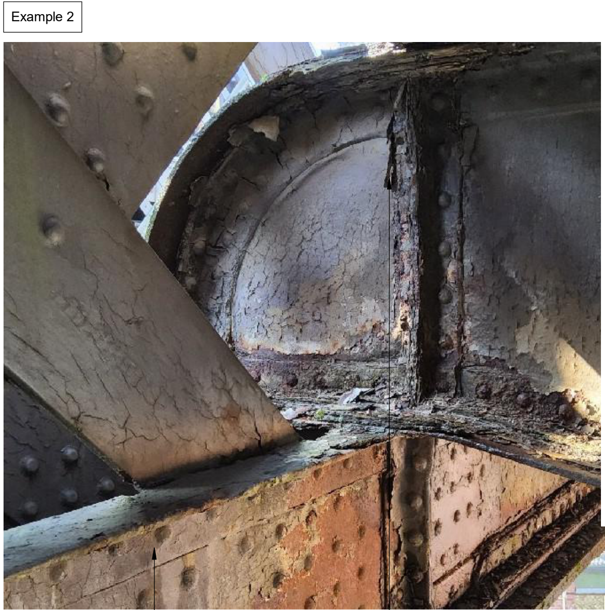
Lattice girder bottom chord Corrosion typically where transverse beam extends beyond weathering protection of deck plate
