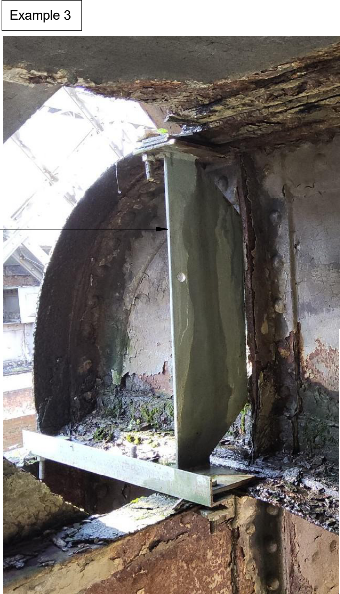
Lattice girder bottom chord Corrosion typically where transverse beam extends beyond weathering protection of deck plate
