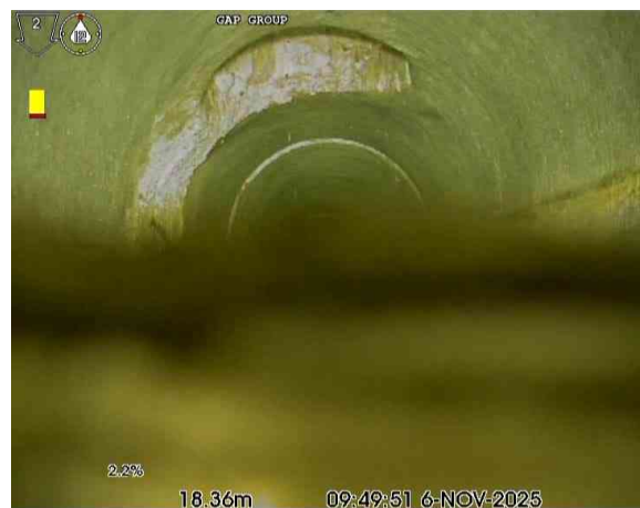
4, 00:03:05, 18.36 m Junction at 12 o'clock, 150mm dia
