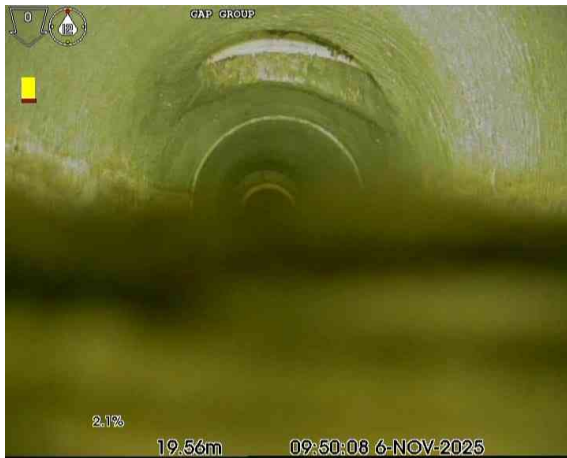
5, 00:03:22, 19.56 m Junction at 12 o'clock, 150mm dia
