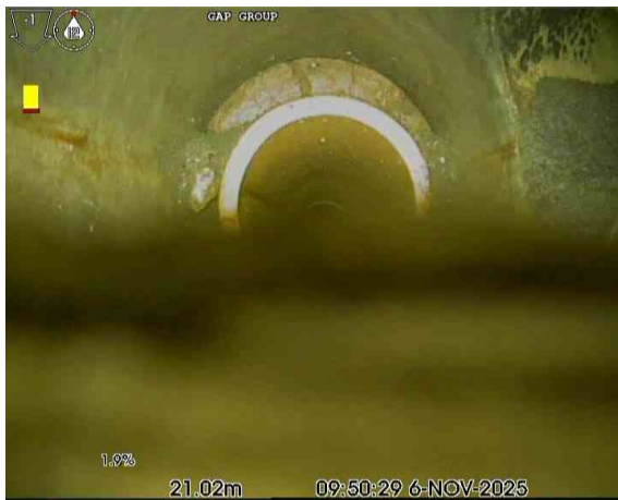
7, 00:03:43, 21.66 m Pipe size changes, new size(s), 150mm high
