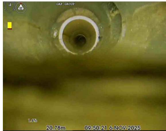
6, 00:03:35, 20.78 m Junction at 3 o'clock, 150mm dia
