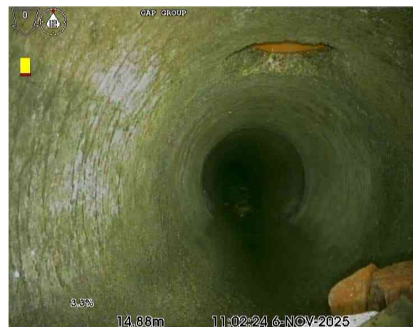
4, 00:02:31, 14.88 m Junction at 12 o'clock, 100mm dia
