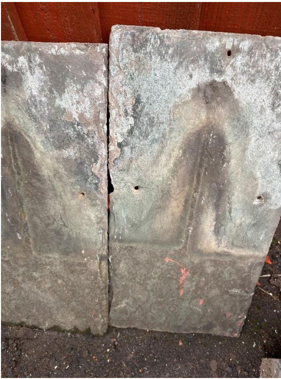
Figure 2: Salvaged Roof Tiles to match existing
