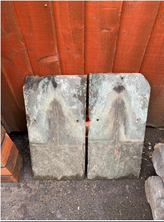
Figure 1: Salvaged Roof Tiles to match existing
