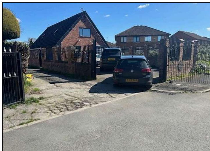
View of application property from Victoria Terrace
