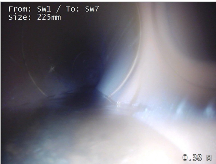
Junction at 2 o'clock, diameter 150mm
