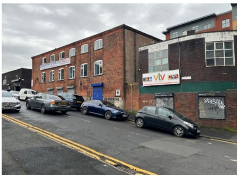
View of application building from Stocks St
