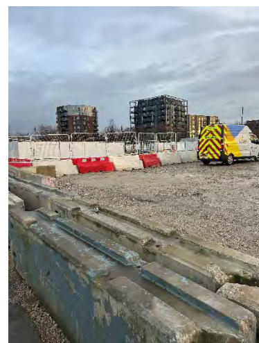
Figure 6 - Southern site section showing site use as a storage area for adjacent construction works
