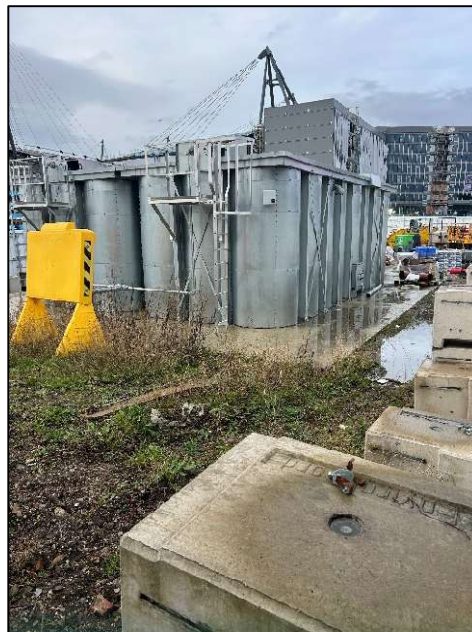
Figure 10: Tanks in the southeastern site section
