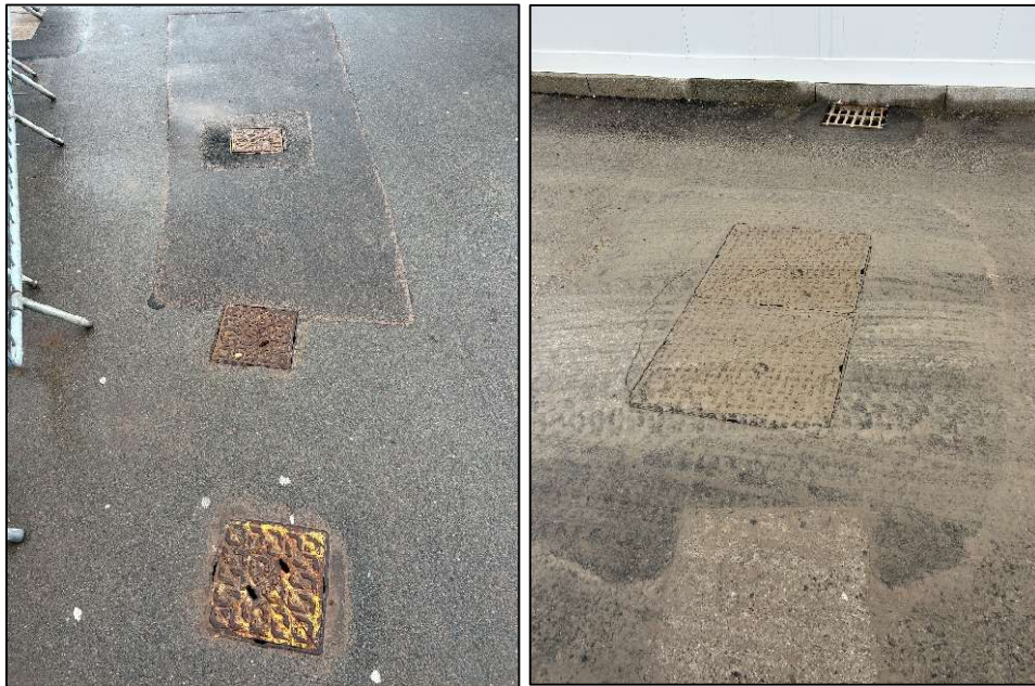
Figure 9: Gas covering to the west of the site (left) and drainage covering to the south of the site
