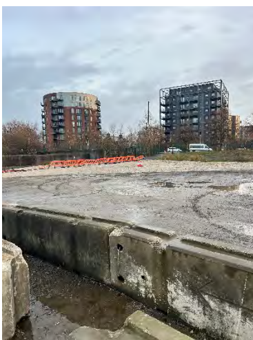
Figure 5 – Site condition facing northeast showing ground underfoot comprising 6F2 and Asphalt
