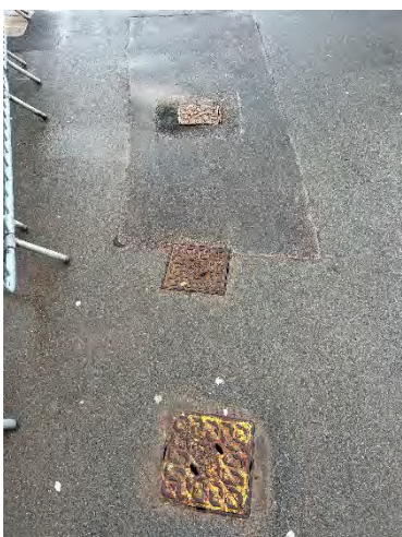
Figure 13 – Gas main coverings west of the site
