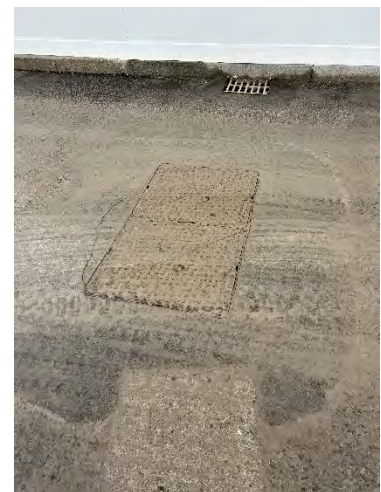
Figure 12 – Sewer covering to the west of the site
