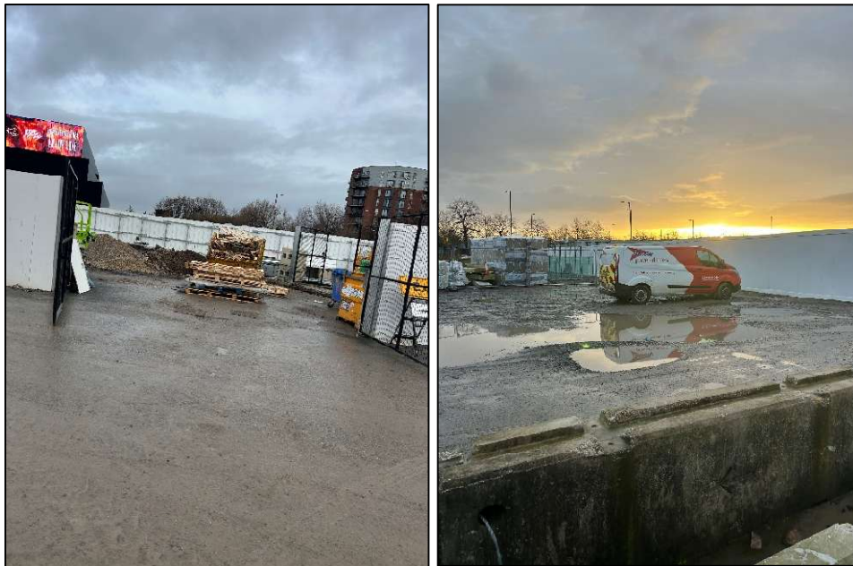
Figure 8: Photographs showing the site compound facing north (left) and southeast (right)
