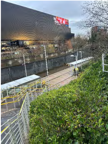
Figure 7 – Metrolink cutting to the north of the site facing north east with the Co-op Live arena in the background
