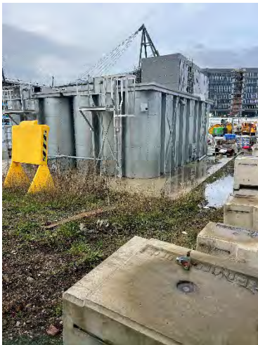
Figure 9 – Industrial land use in the southern site section
