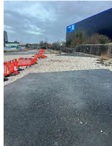
Figure 2 – Present site condition with the Metrolink cutting, Ashton Canal and Co-op Live arena in the background facing northwest
