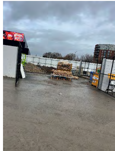
Figure 8 – Southern site section currently in use as a storage / stockpiling area facing north
