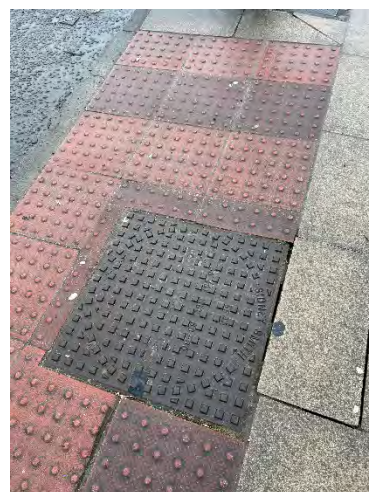
Figure 14 – Sewer covering to the east of the site
