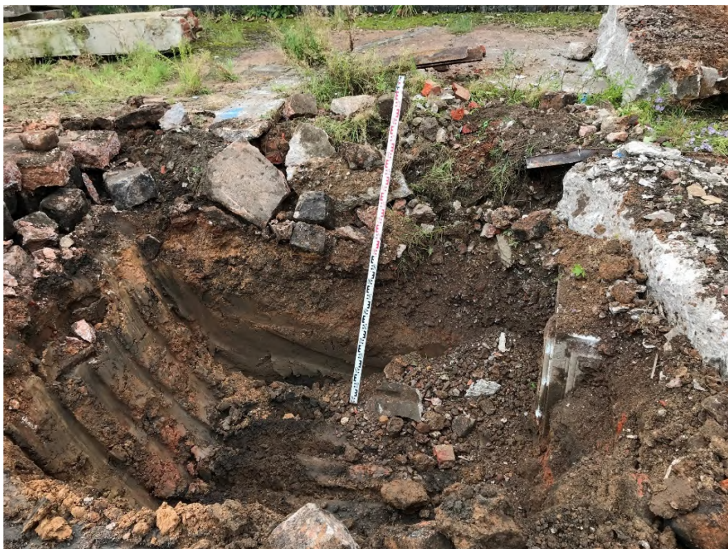
Photo No. I3: TP304
