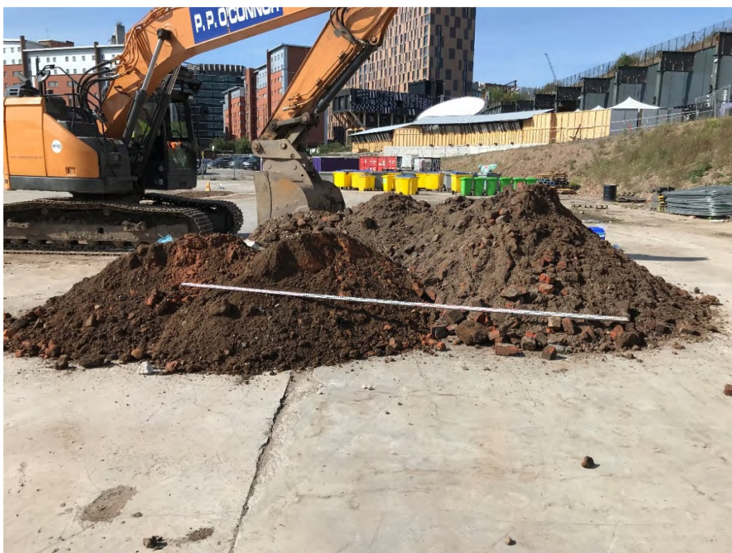
Photo No. 40: TP31 I Arisings
