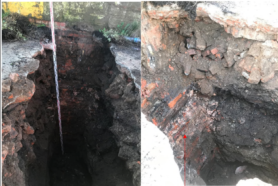
Stepped brick masonry
