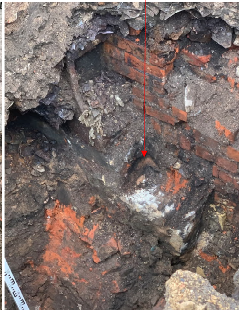
Hog's-back beam on padstone
