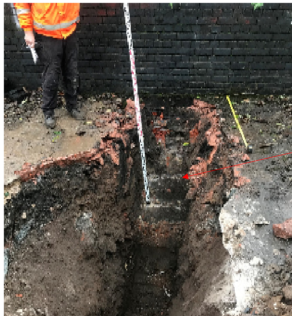
Concrete footing stepping out
