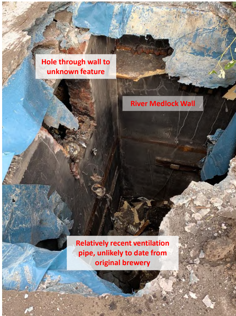
Photo into basement looking north
