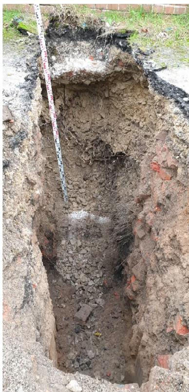
Plate No. 17: PP TPI09A footing founded on sandstone
