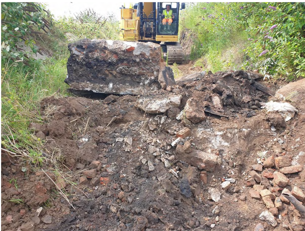
Photo No. 11: TP403 Arisings
