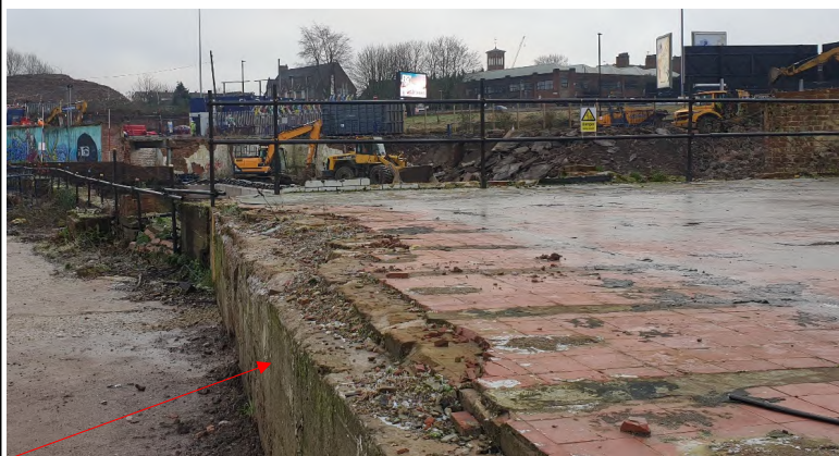
Raised Concrete 'podium', Culvert entrance. Formed part of historical building
