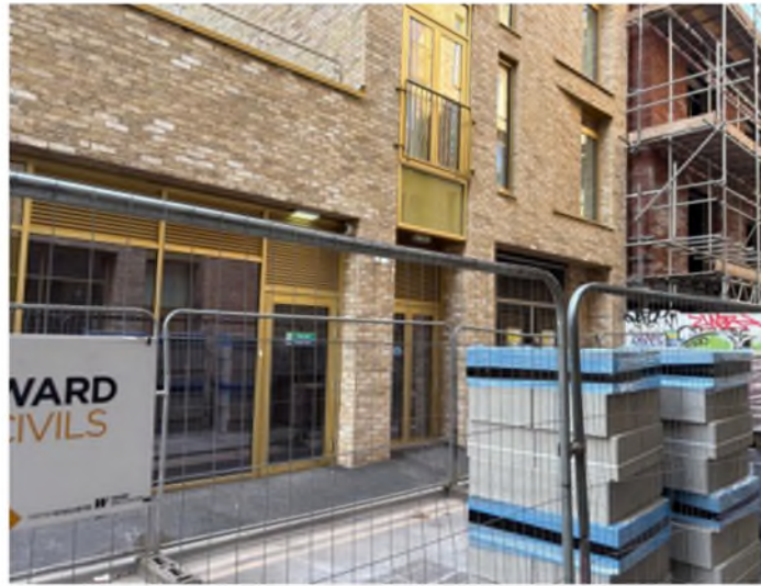
Louvres installed on Spear Street elevation
