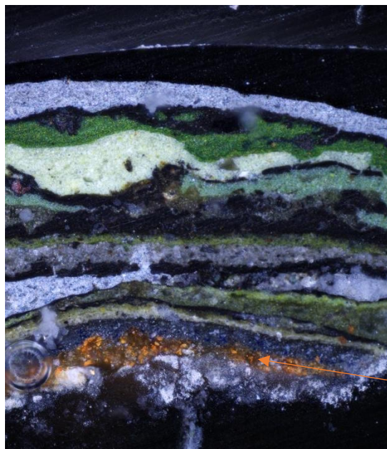
Figure 16: Sample 05B (200x mag) showing use of red lead primer beneath the grey undercoat.
