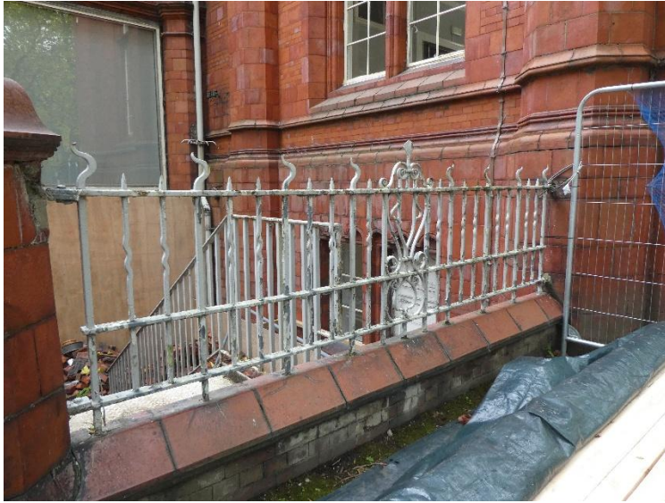
Figure 11: image of the east end railings with later fire escape behind
