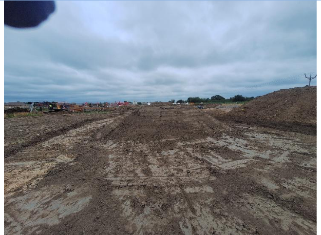
Photograph 2 – TS5 Front view
