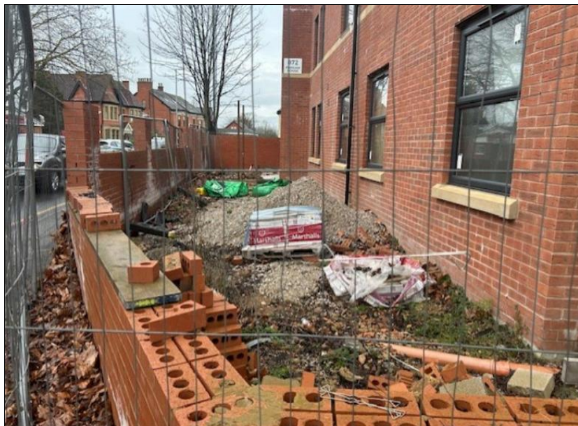
View of front yard area
