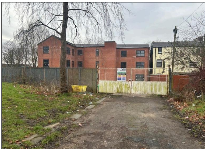
View of rear of application site from Tudor Avenue
