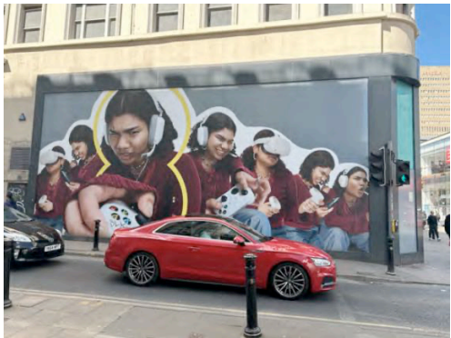
existing shopfront photograph
