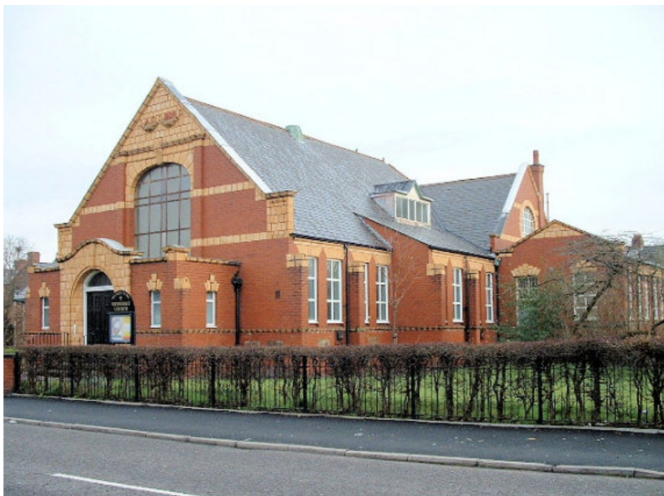
Figure 15- Manley Park Methodist Church, Whalley Range
