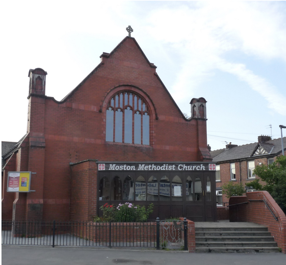
Figure 14- Streetfold United Methodist Church, Moston
