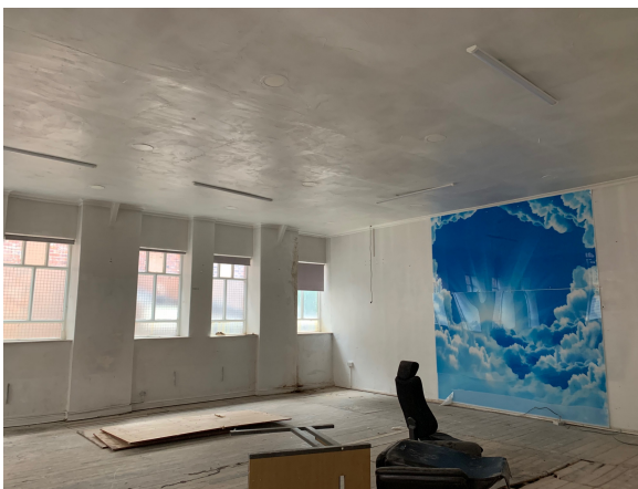
Figures 11 and 12- first floor rooms
