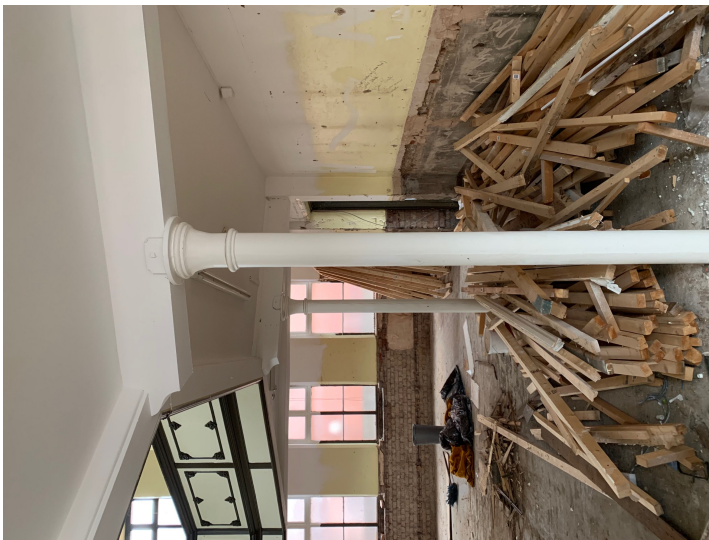
Figure 9- columns and beams to transverse galleries Figure 10- columns/beams to north gallery
