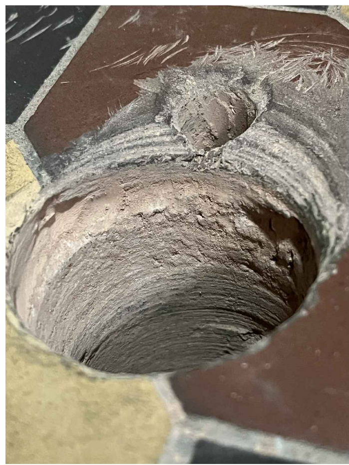
EXISTING MOSAIC FLOOR TILE BEDDED IN CONCRETE.
