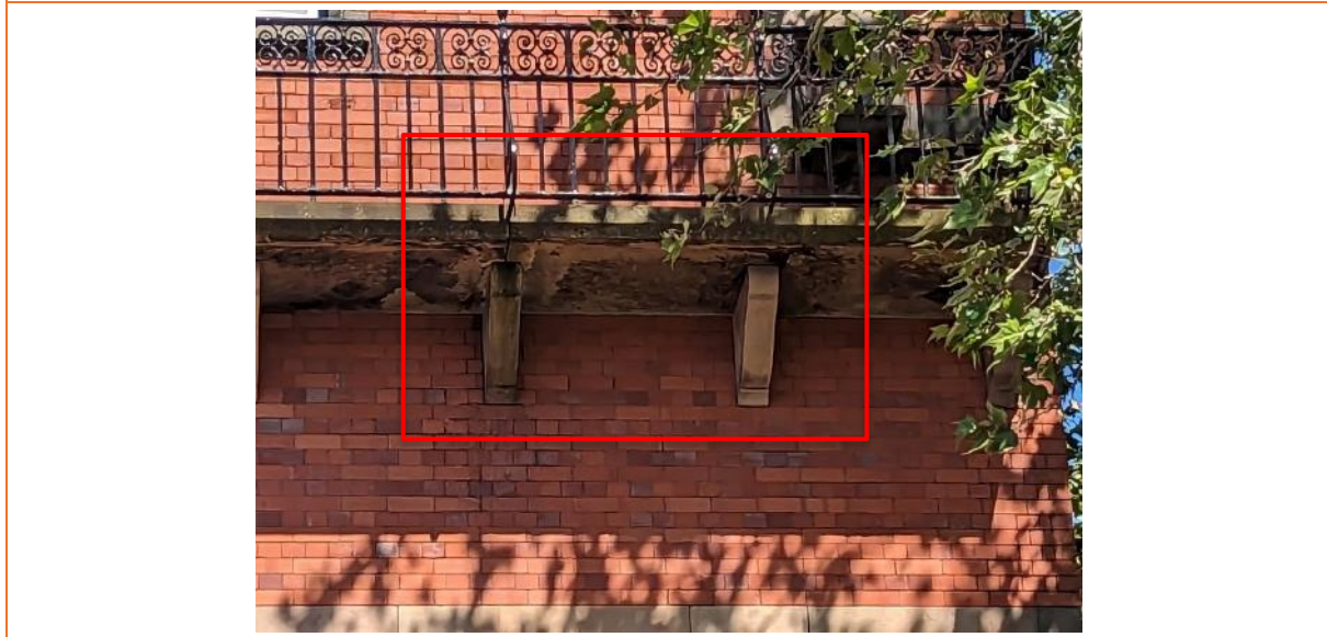
PLATE 3 SHOWING STONE BALCONIES
