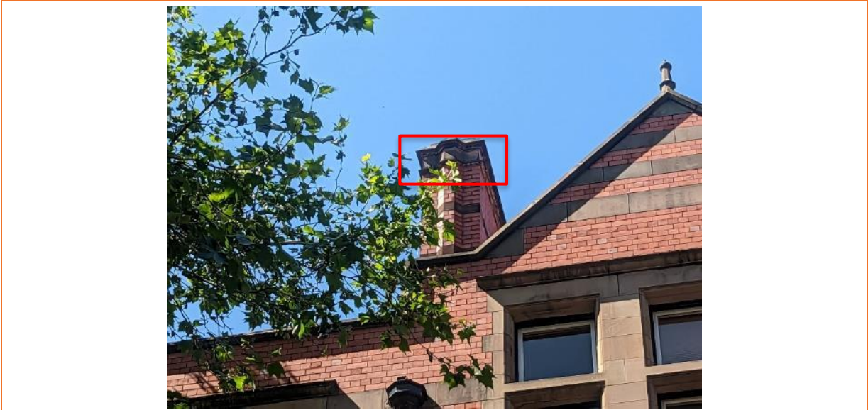
PLATE 5 SHOWING THE SOUTHERN CHIMNEY STACK
