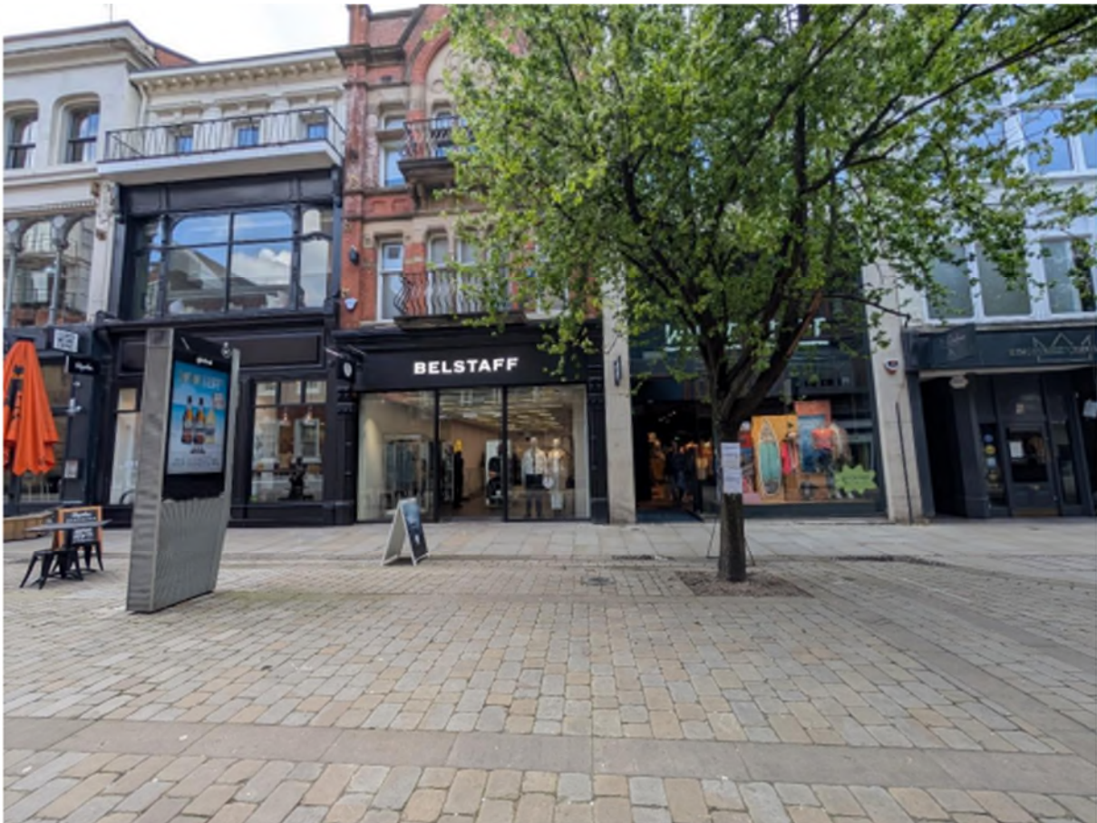
(Figure 14: Application site along King Street, within Primary Shopping Area/Retail Core)
